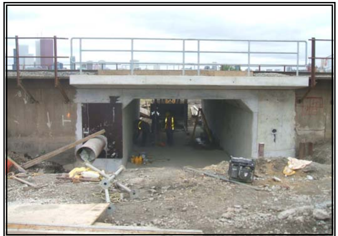
Looking West Under Bala Underpass
