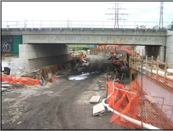
Looking South Under New Don River Bridge
