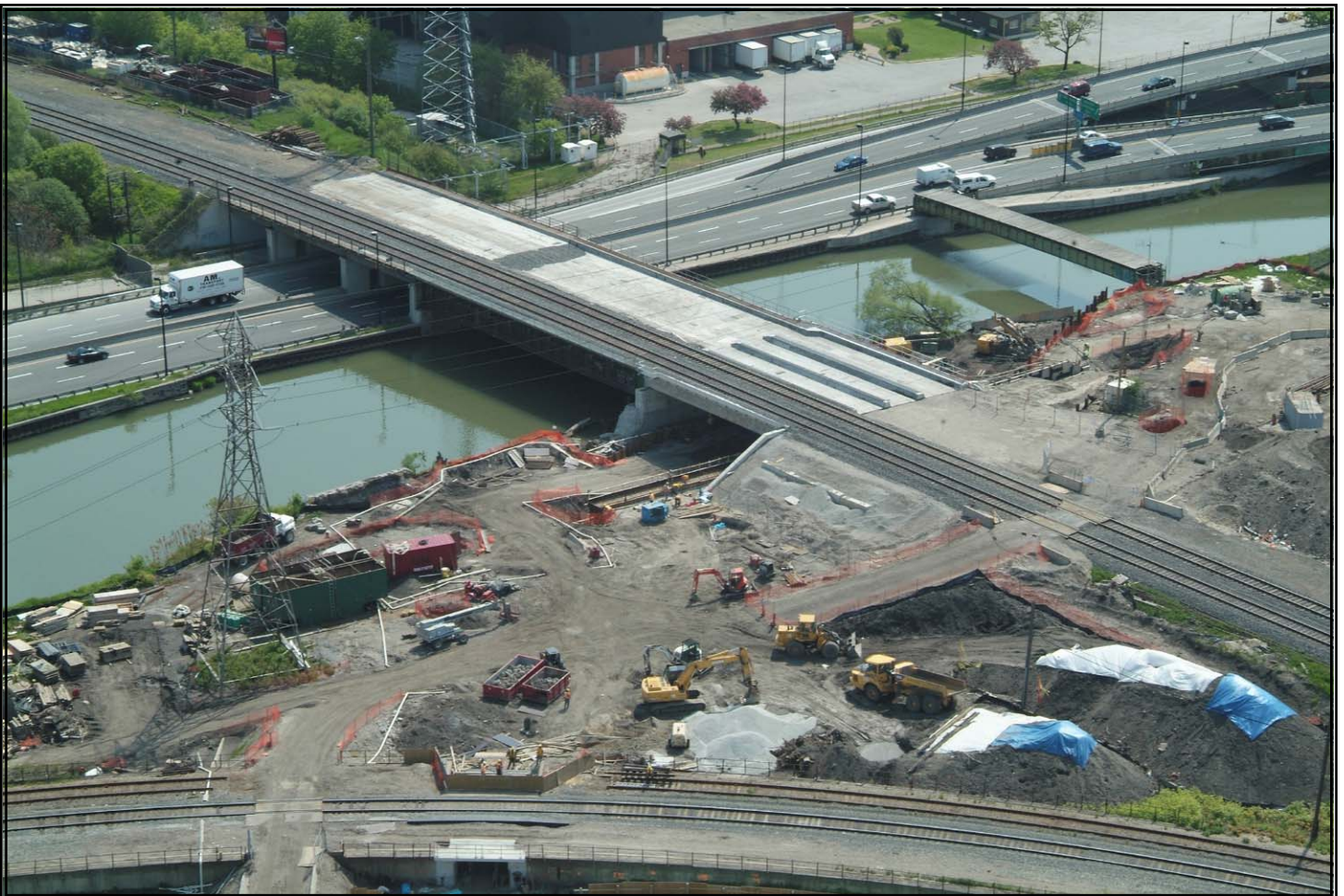
Northern Span of New Don River Bridge and Bala Underpass
