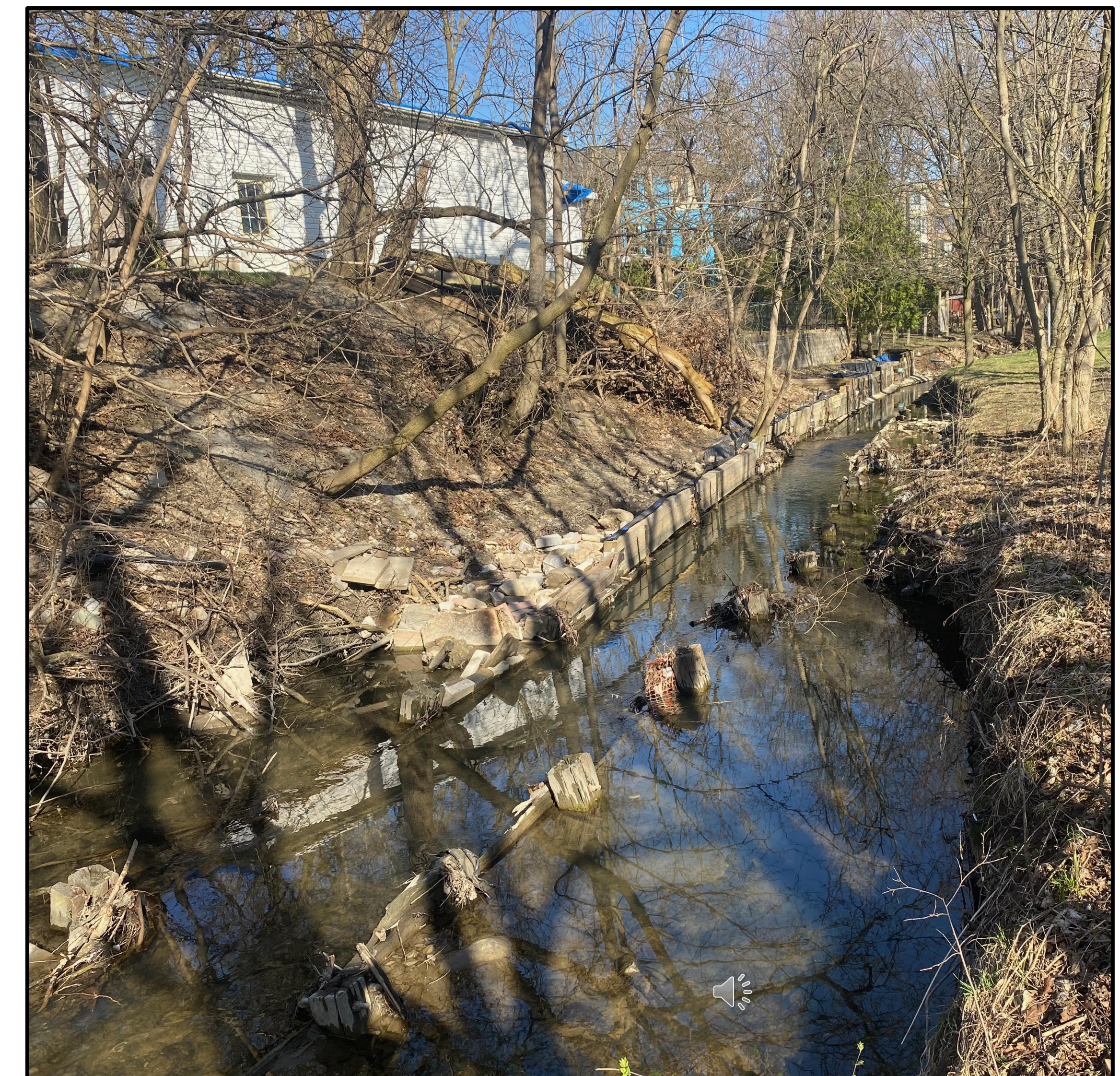
Bank erosion impacting adjacent residential properties
