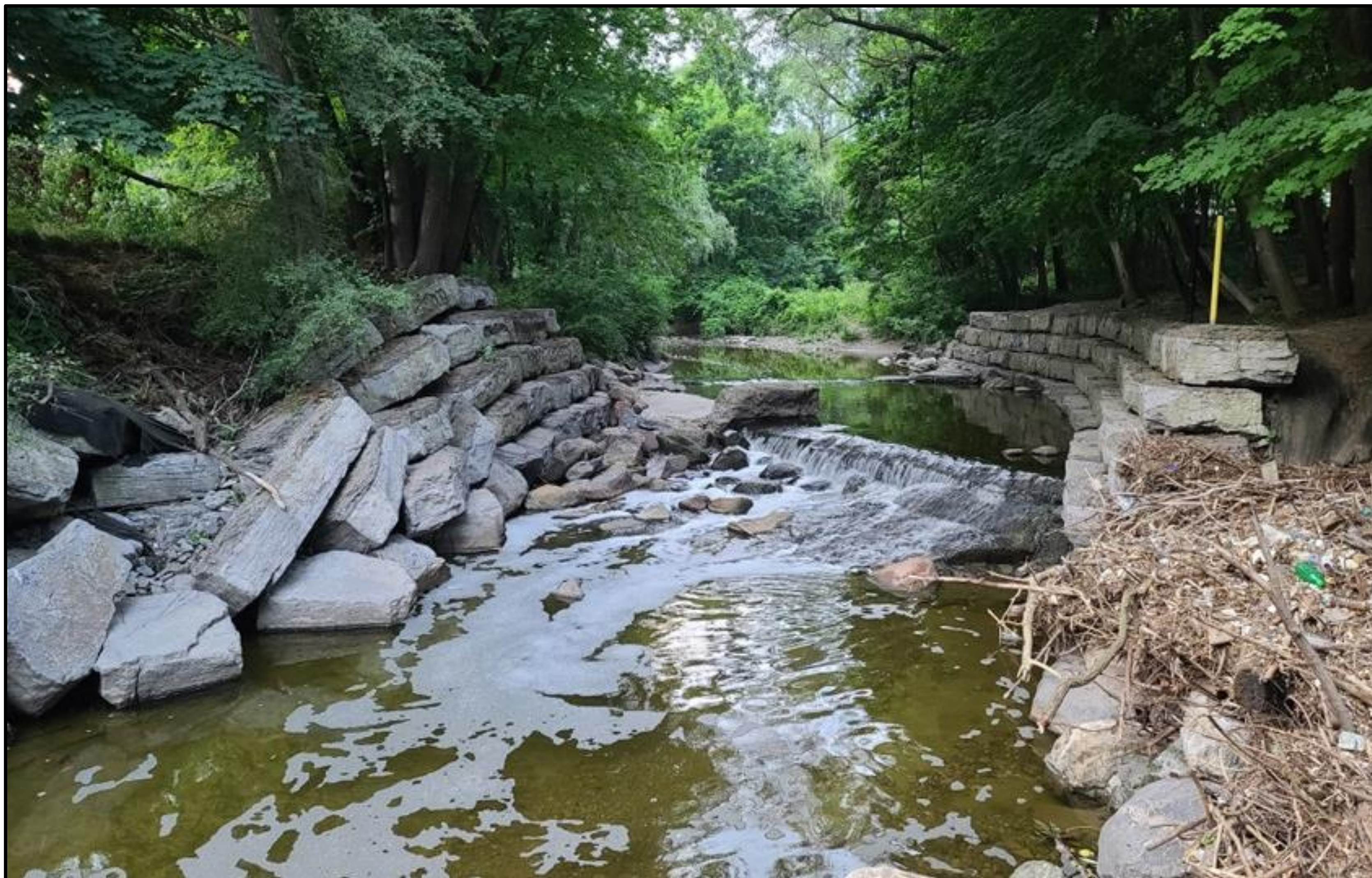
Exposed Sanitary Sewer and Failed Armourstone Retaining Wall (August 2020)
