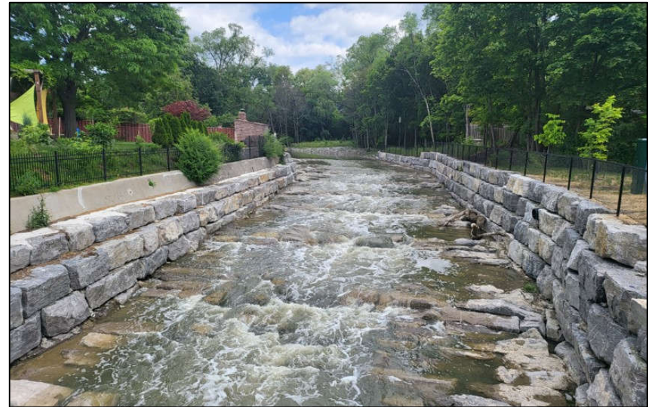
Armourstone Bank and Bed Control (June 2023)
