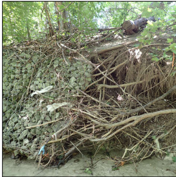
Undermined gabion baskets and heavily eroded channel banks
