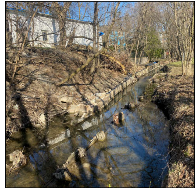
Bank erosion impacting adjacent residential properties
