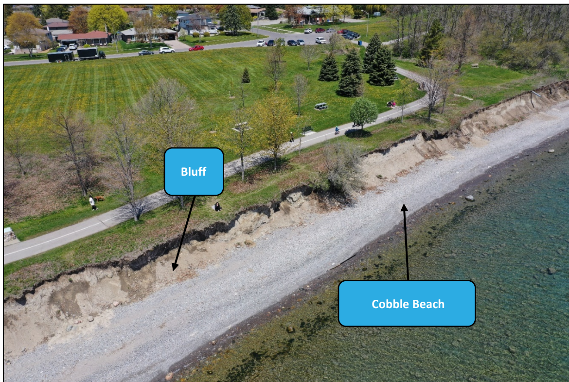
Figure 5. Aerial view of the shoreline at the eastern end of Lake Driveway East. Source: TRCA, 2021.
