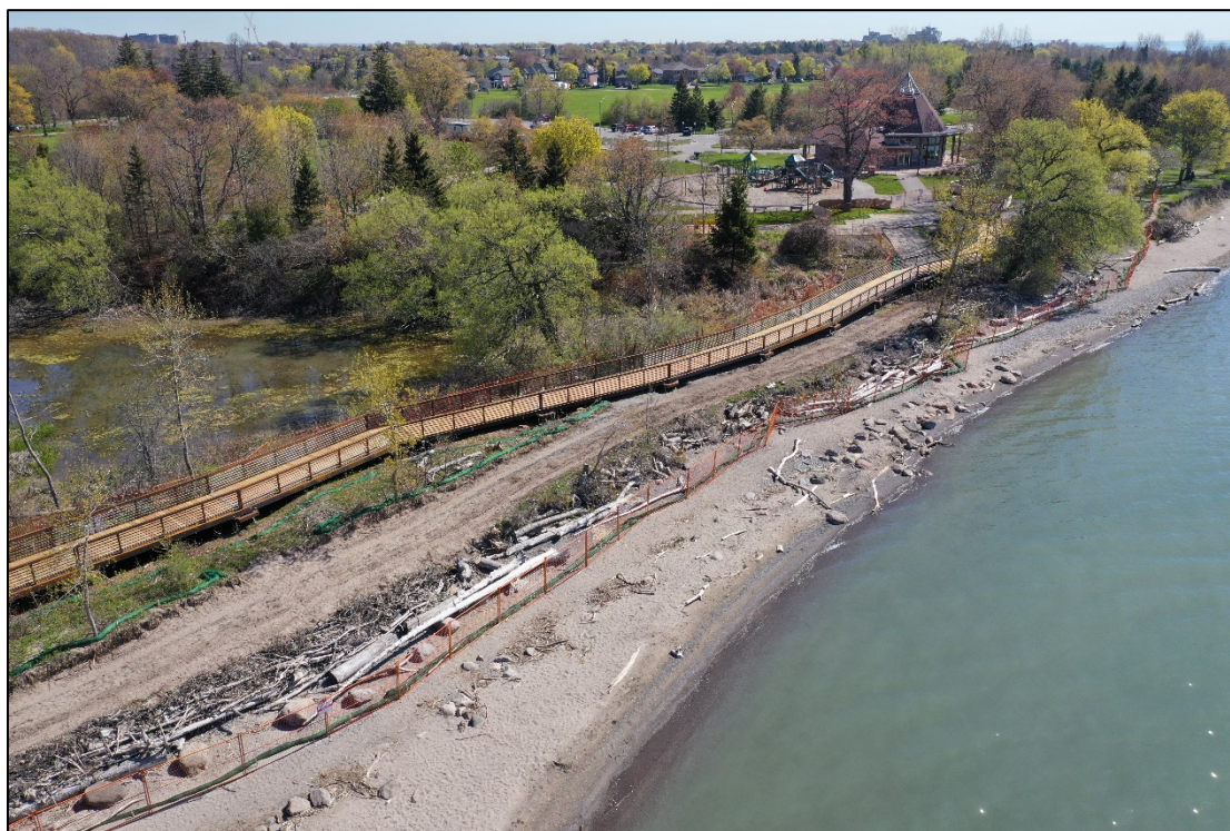
Figure 9. Part of the Duffins Creek Boardwalk. Source: TRCA, 2022.
