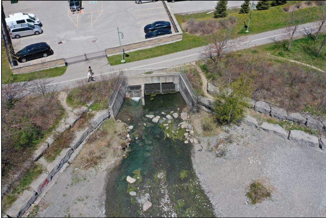
Figure 27. Stormwater outfall located near the Ajax Water Supply Plant. Source: TRCA, 2021.
