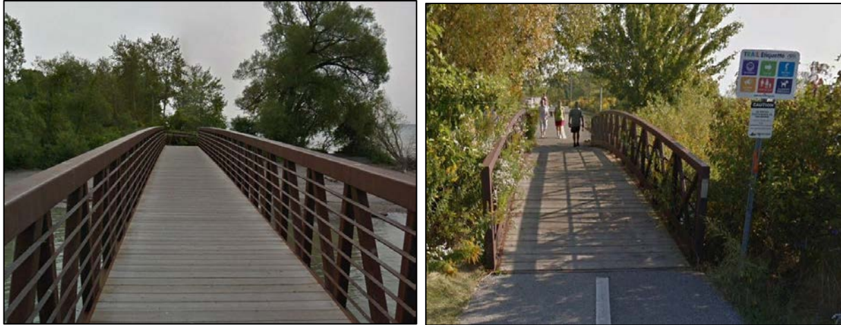
Figure 17. The boardwalk at Duffins Creek and the pedestrian crossing located west of the Ajax Water Supply Plant. Source: Google Earth, 2021.
