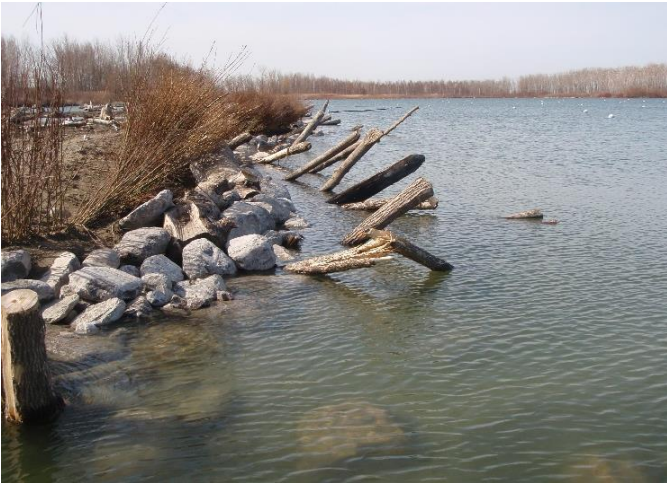
Figure 64: Live stakes, nearshore boulder shoal and anchored log fringe of the created wetland berm in Embayment C, South Shore. (TRCA 2011)
