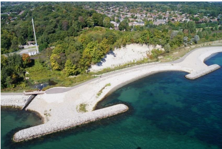
Figure 4: Port Union Phase II detail: Armourstone headland, cobble beach, and Adam's Creek mouth (TRCA 2013)
