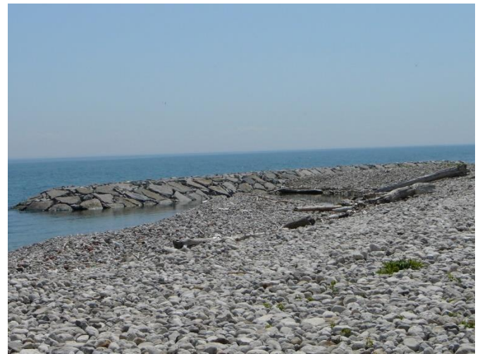
Figure 5: Cobble beach natural sorting and recruitment of woody debris at Port Union Phase I (TRCA 2009)
