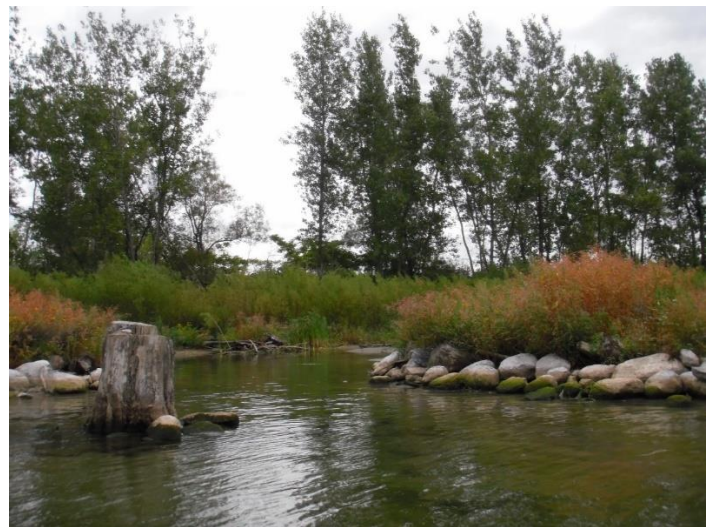
Figure 56: Woody material and boulders armour the created islands, giving way to the vegetated backwater channels of Embayment A. (TRCA 2013)
