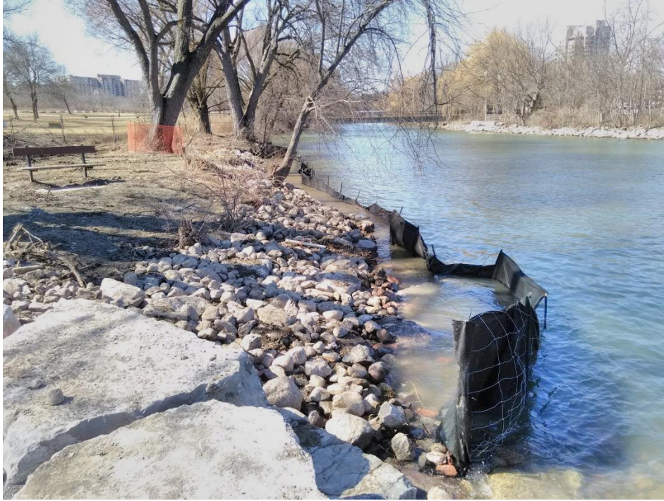
Figure 26: Shoreline restoration work underway at Marie Curtis Park's Etobicoke Creek. (TRCA 2017)
