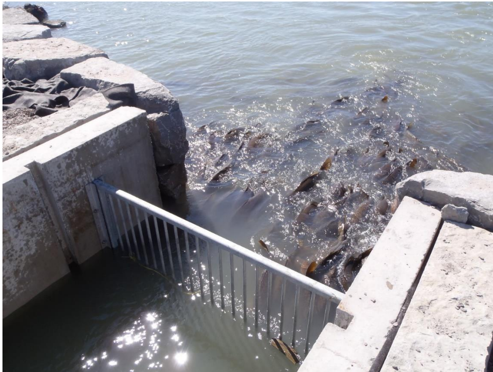
Figure 84: Common Carp attempting to enter Cell 1 from Cell 2 in Spring 2011, after the water control stop logs were removed. (TRCA 2011)
