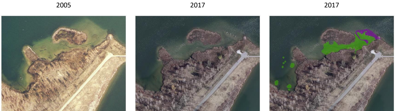
Figure 77: Embayment C South East Footpad project before (left) and after (centre). Project polygons are shown to the right. (Photos: First Base Solutions 2005; City of Toronto 2017)
