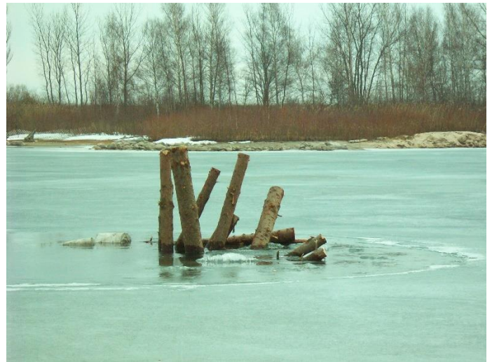
Figure 70: Log Piles, Log Tangles, and Boulder Clusters left on ice and melting through ice of Embayment C North East Shore. (TRCA 2010)
