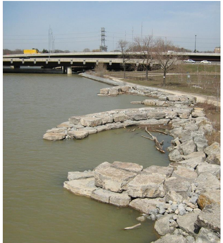
Figure 21: Estuary hooks in high spring flows. Woody material has been captured in back eddy pools. (TRCA 2008)
