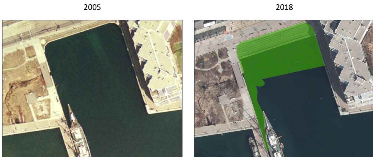
Figure 47: Spadina Slip Wavedeck Project before (left) and after (right), shown with project polygons. (Photos: First Base Solutions 2005; City of Toronto 2018)
