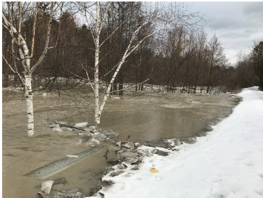
FIGURE 3-25: PICKERING DYKE DURING ICE JAM FLOODING – MARCH 15, 2019. WATER AGAINST THE WET SIDE OF THE DYKE
