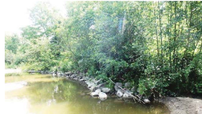
Creek bank erosion repair.
