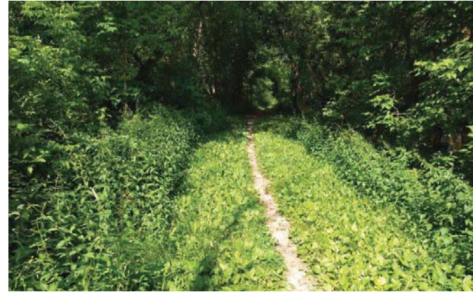
Narrow dyke crest and tree growth on dyke.
