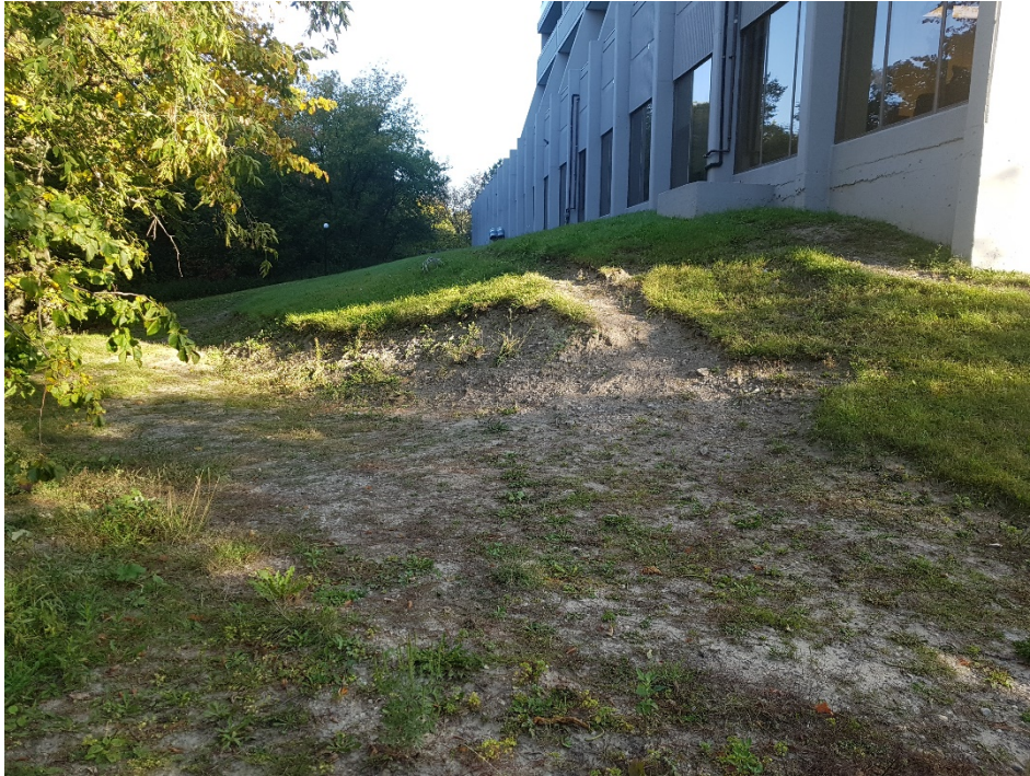
M20- Ajax Dyke Tie-in at Condo Building at 92 Church St S
