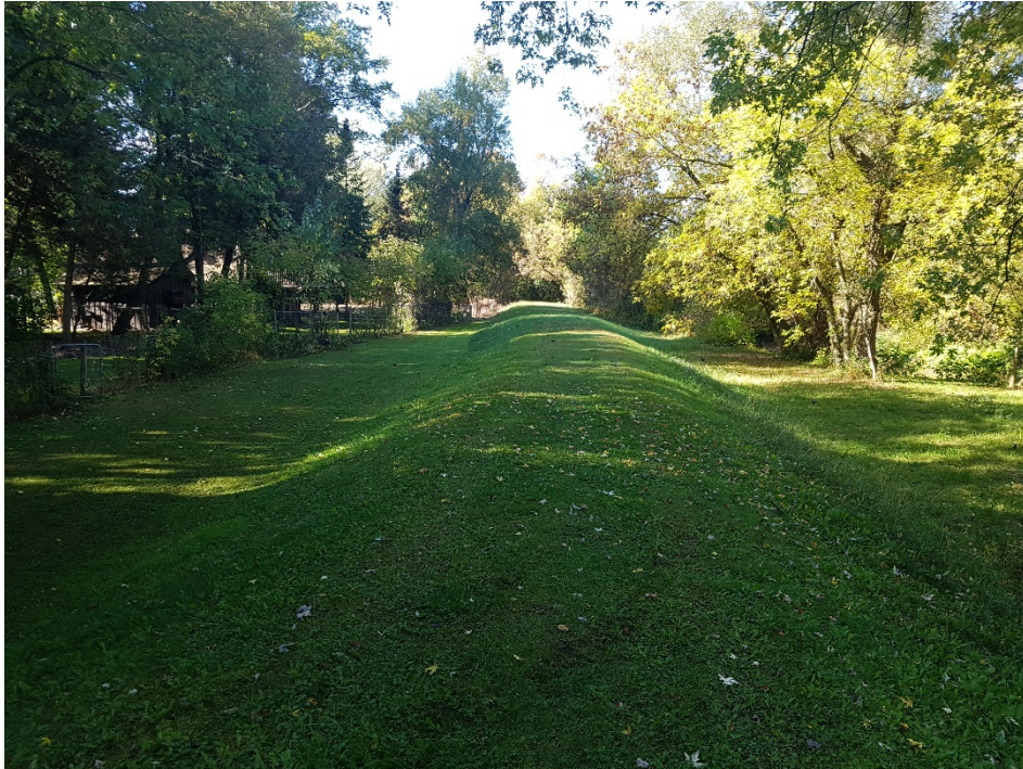
M3-Pickering Dyke 100 m to 200 m East of Brock Rd
