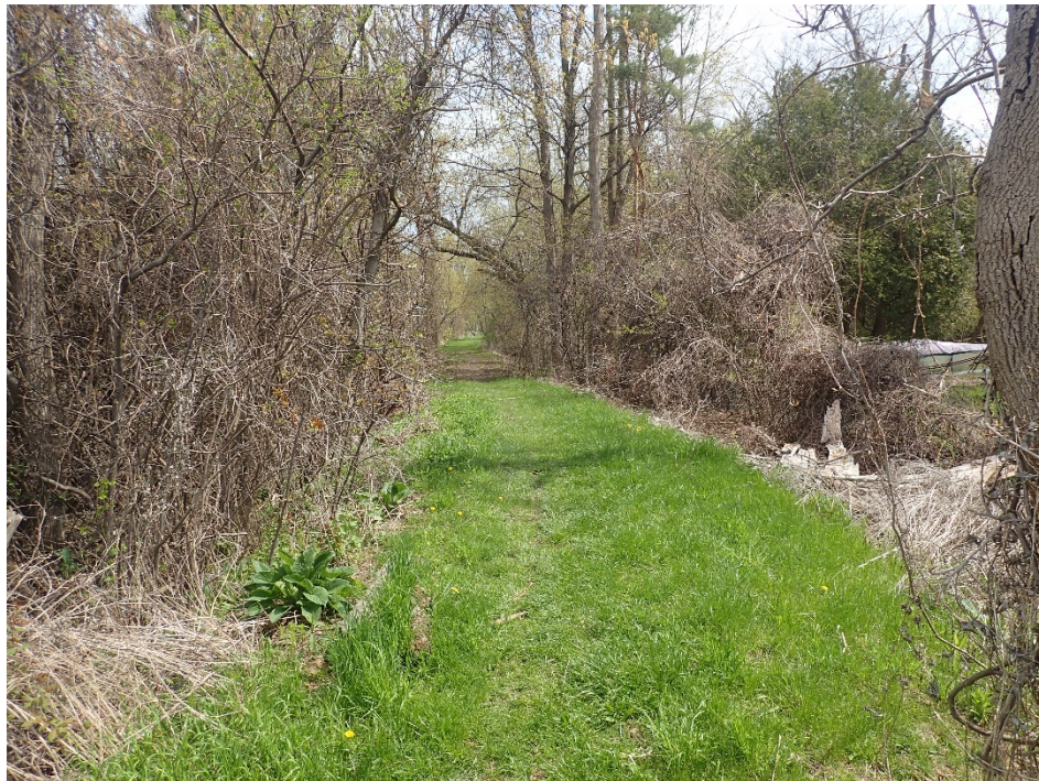
M2-Pickering Dyke Approximately 50 m East of Brock Rd
