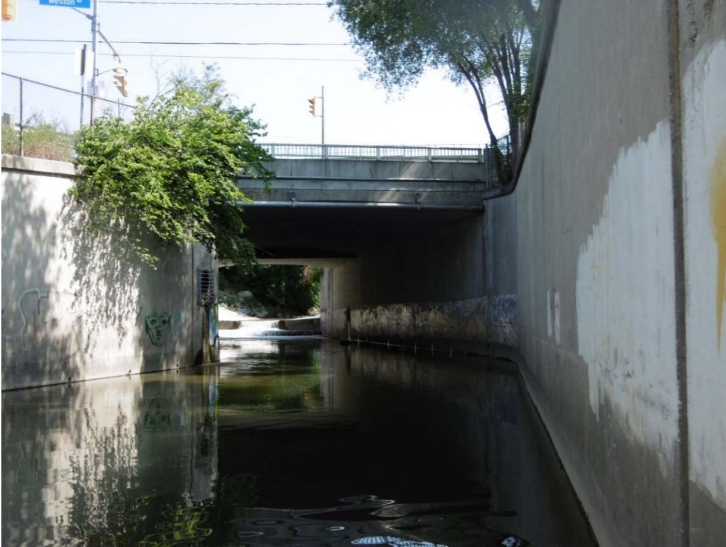
Photograph 6.2. Downstream of Weston Road Existing Crossing
