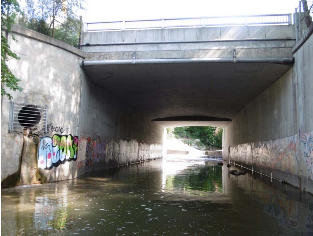
Photograph 6.1. Weston Road Existing Crossing
