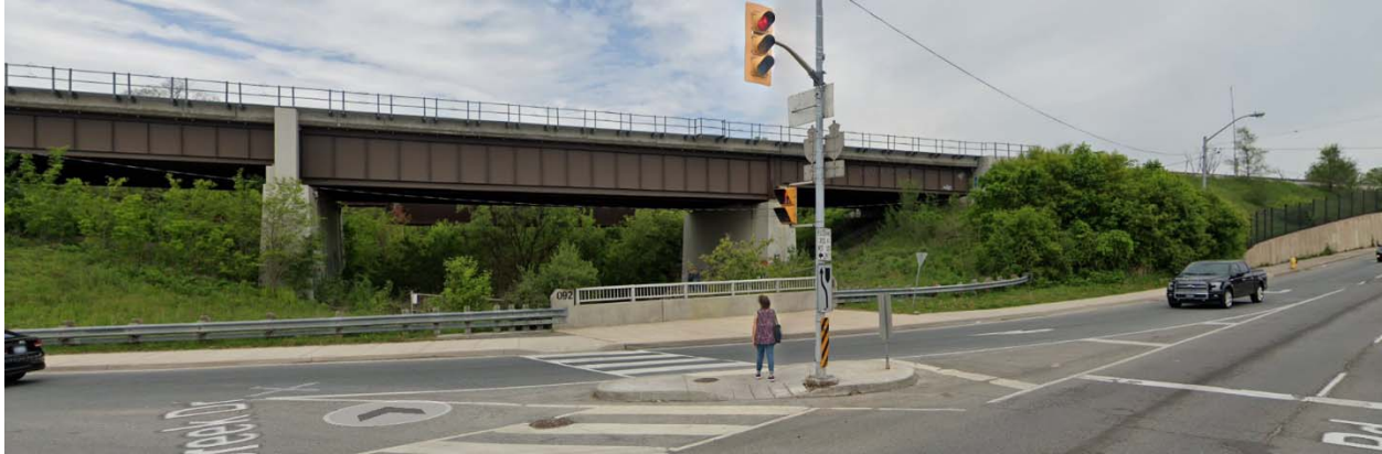
Photograph 6.4. Parapet Wall on Upstream Side of Weston Road Crossing
