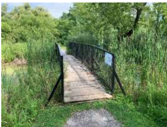
Figures 45 & 46: (left) View of bridge looking south from Black Creek Trail, (right) Detail view of wood plank bridge deck and steel railing system, (Source: MHBC, 2019)
