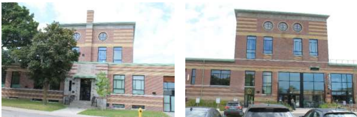
Figures 50 & 51: (left) View of east façade of former incinerator building, looking west from Symes Road, (right) View of west façade of former incinerator building looking east from parking lot. (Source: MHBC, 2019)
