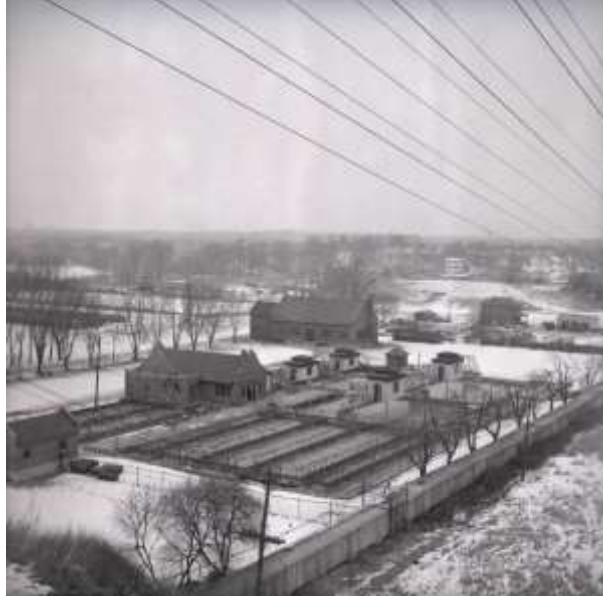
Figure 15: Historical photo of the Rockcliffe Sewage Plant, 1954. (Source: Toronto Public Library)
