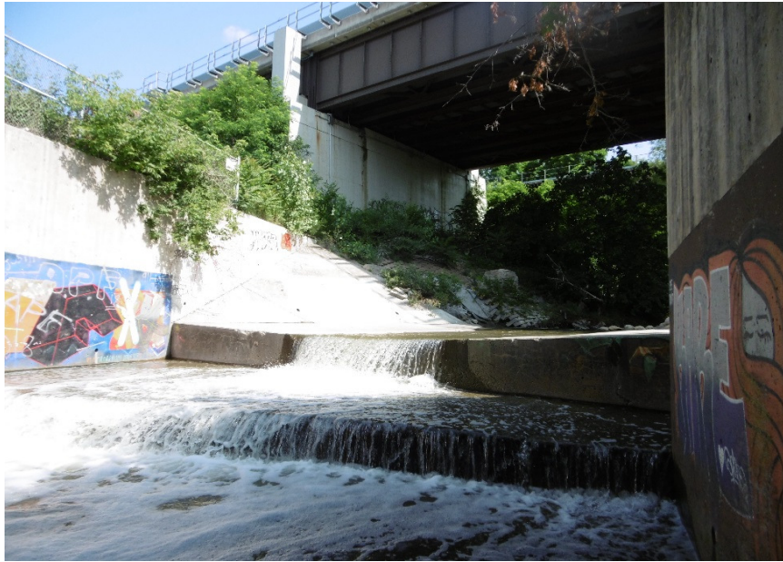
Description of Photo: Drop structure
