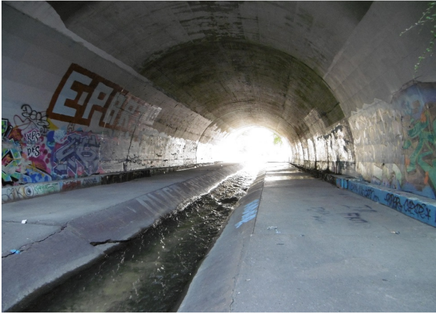
Description of Photo: Inside
