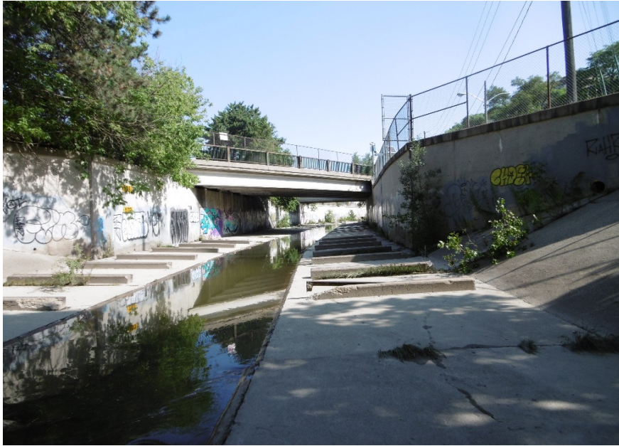
Description of Photo: Downstream face of structure
