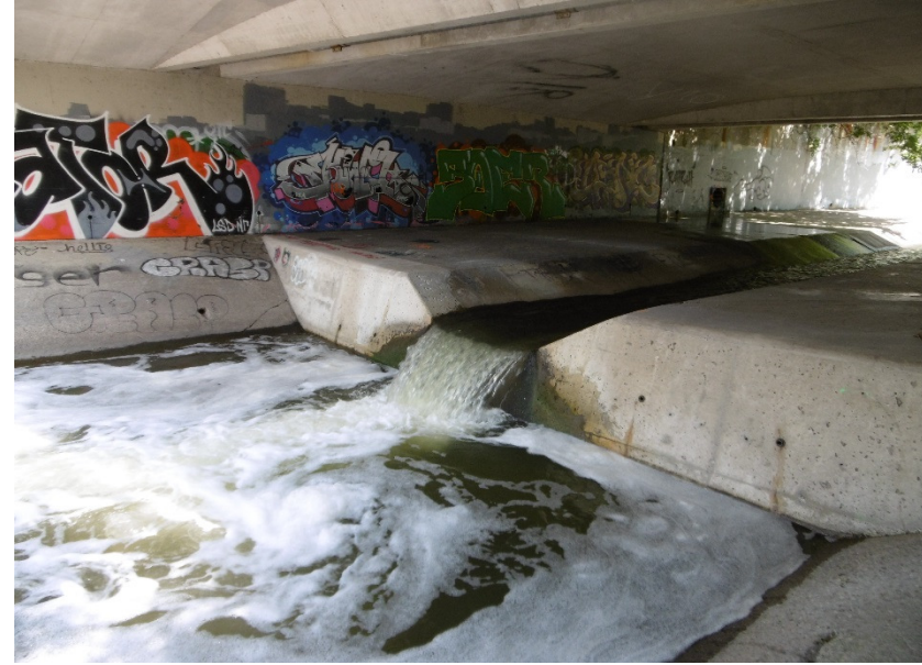
Description of Photo: Drop structure
