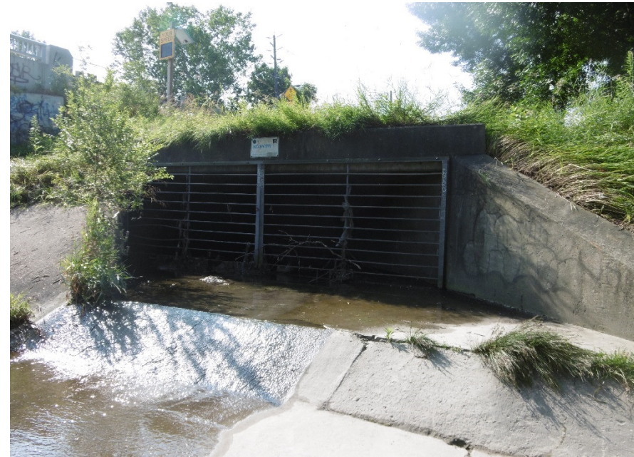
Description of Photo: Storm sewer (downstream)
