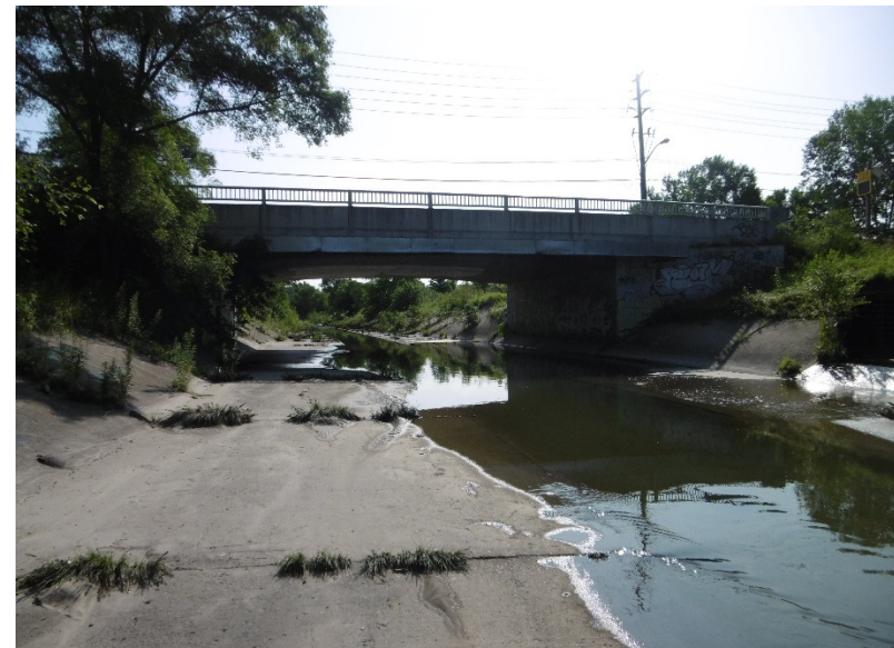
Description of Photo: Downstream face of structure
