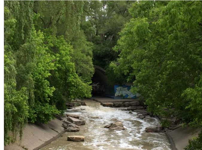
Photo 2 – Downstream side of Jane Street
