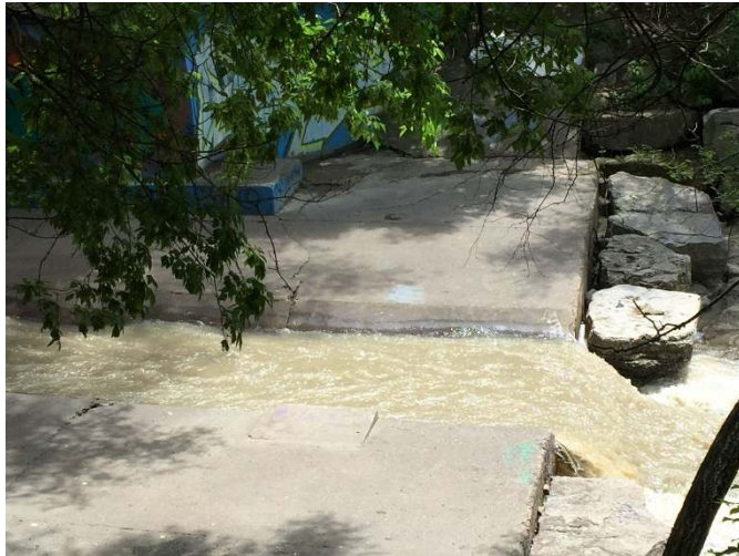
Photo 3 – Downstream side of Jane Street
