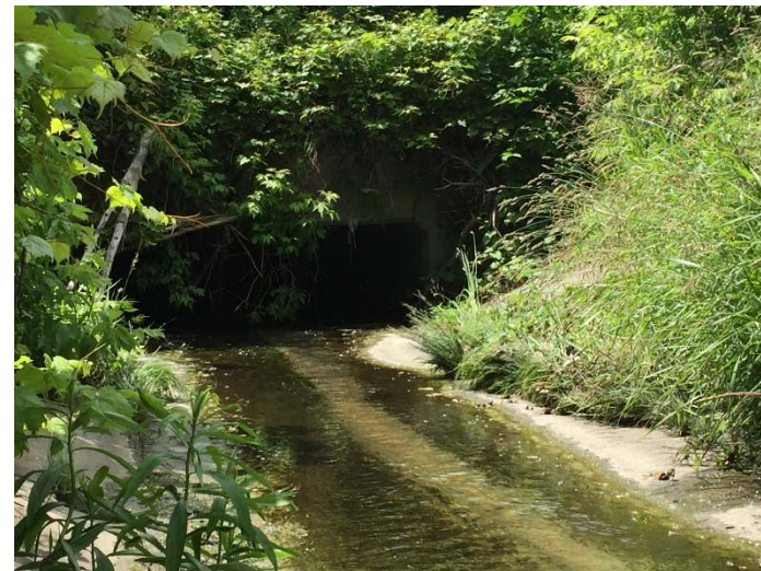
Photo 16 – Symes Road crossing of Lavender Creek
