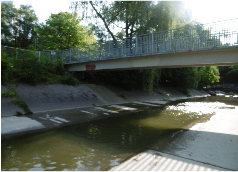
Description of Photo: Downstream structure face
