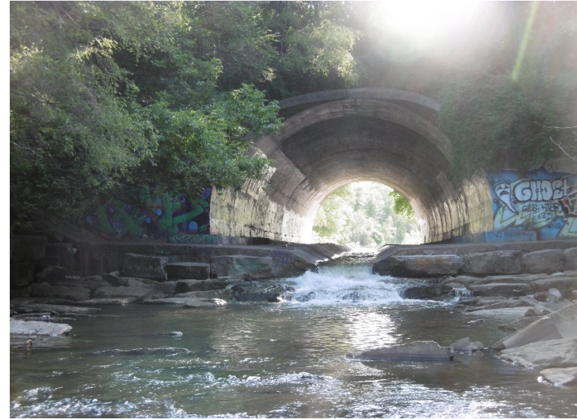
Description of Photo: Downstream structure face
