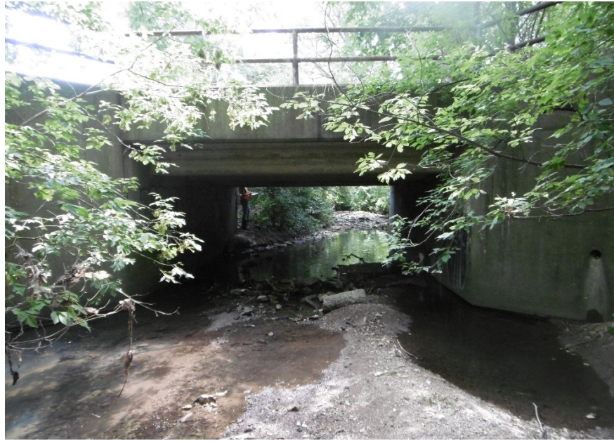
Description of Photo: Downstream face of structure
