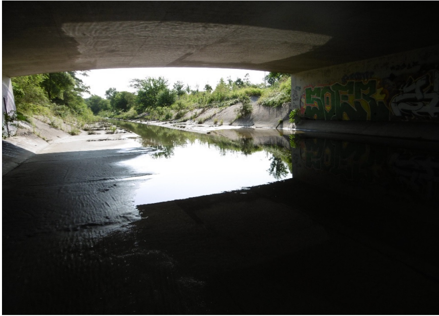
Description of Photo: Inside structure
