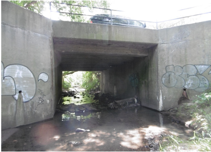
Description of Photo: Downstream face of structure
