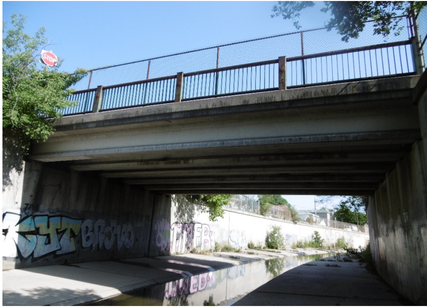
Description of Photo: Downstream face of structure
