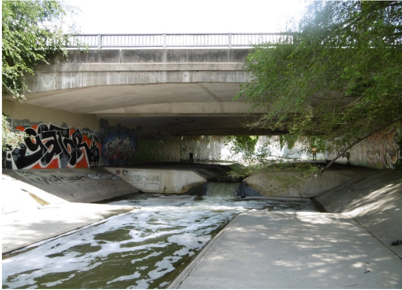
Description of Photo: Downstream structure face
