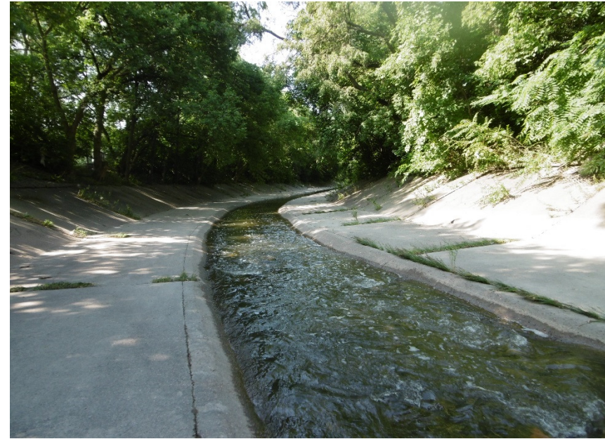
Description of Photo: Storm sewer (downstream)
