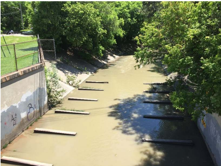
Photo 11 – Flow depth gauge downstream of Alliance Avenue crossing
