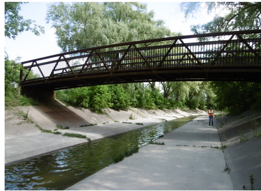
Description of Photo: Downstream face of structure
