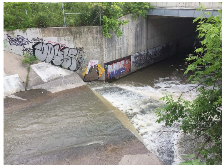
Photo 28 – Upstream of Weston Road
