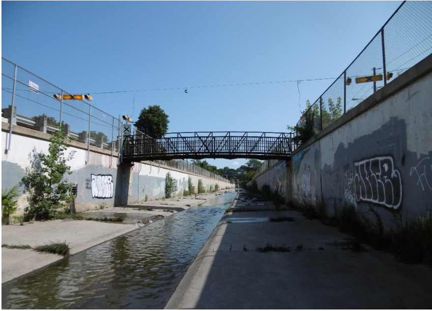
Description of Photo: Downstream face of structure
