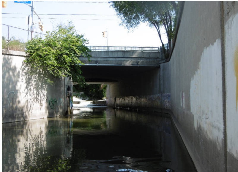
Description of Photo: Downstream structure face
