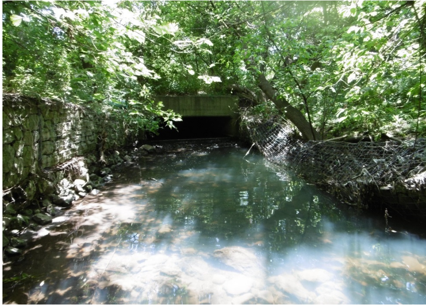
Description of Photo: Downstream face of structure
