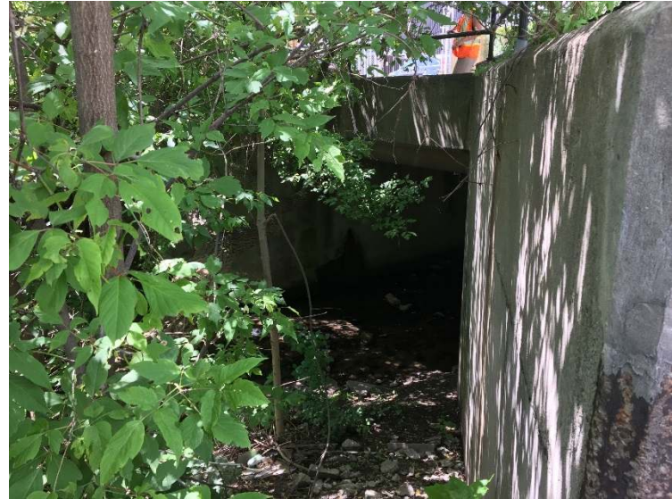
Photo 18 – Lavender Creek driveway crossing
