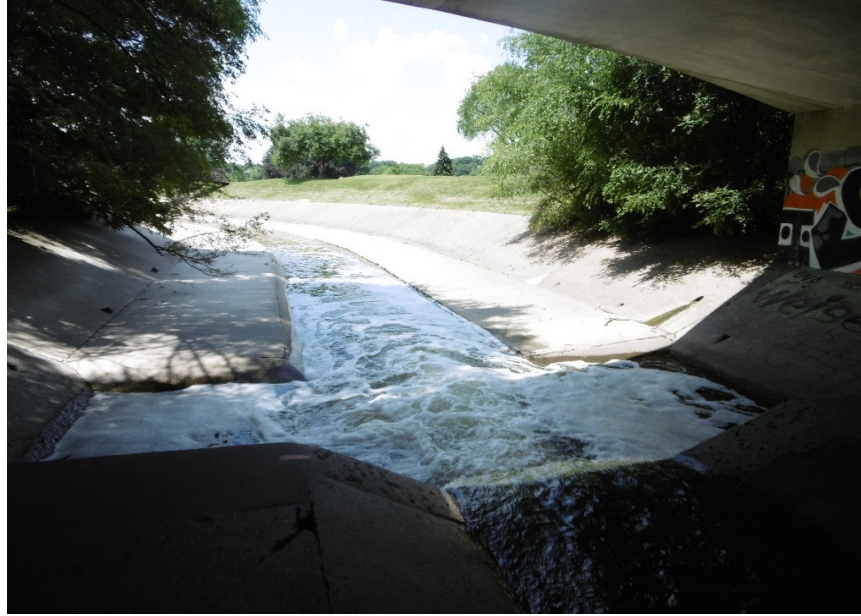
Description of Photo: Inside structure
