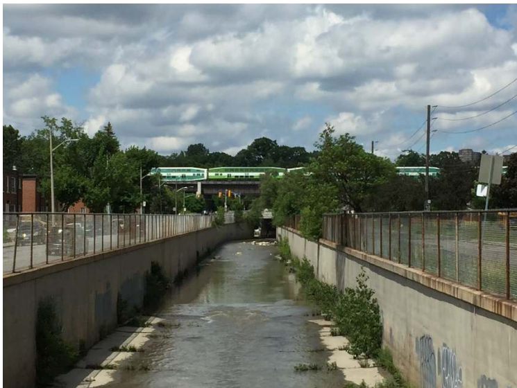
Photo 23 – Looking upstream at Weston Road
