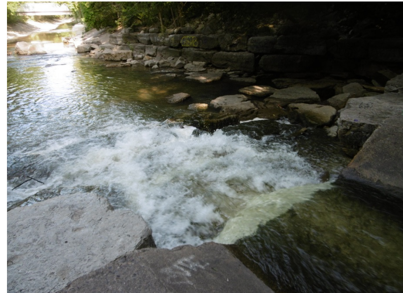
Description of Photo: Drop structure
