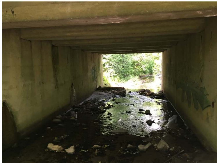
Photo 19 – Lavender Creek driveway crossing
