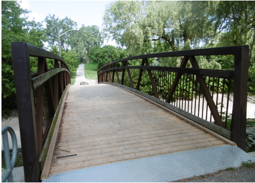
Description of Photo: Path, Railing
