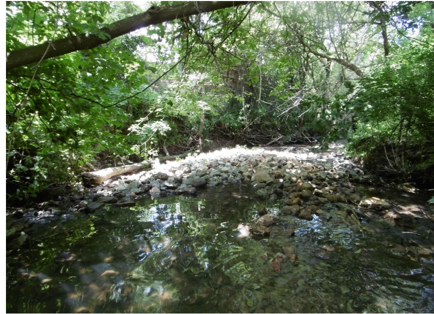
Description of Photo: Downstream channel (note exposed gabion rocks)
