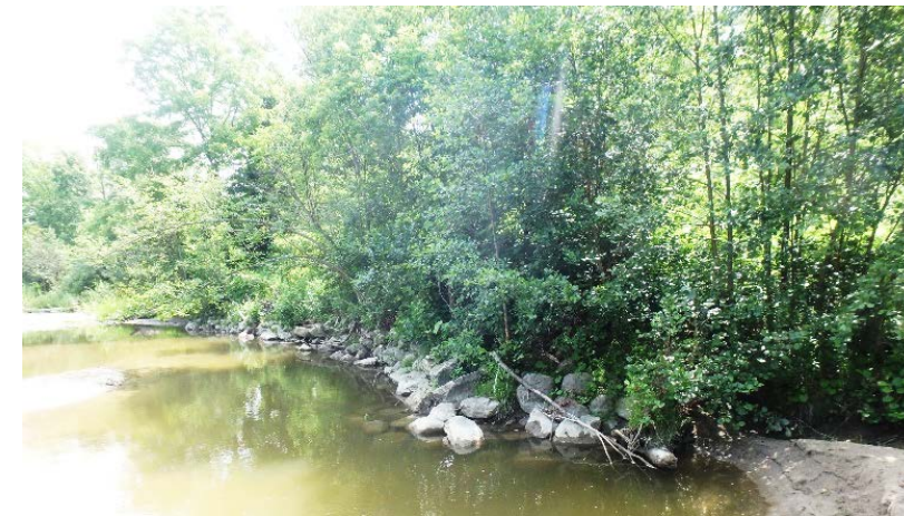
Creek bank erosion repair.
