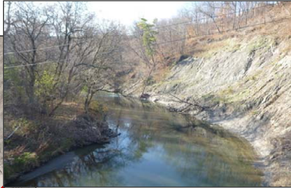
Low west bank and erosion along east river bank
