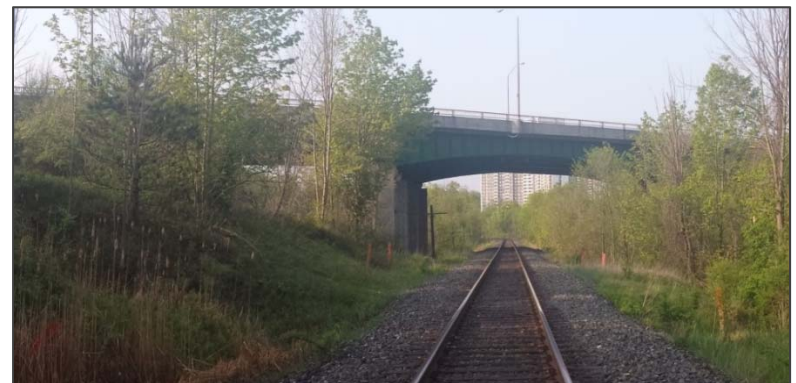
Location of rail line crossing north of Eglinton Ave
