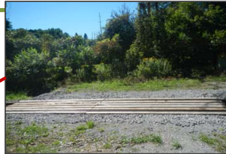
Existing maintenance level crossing
