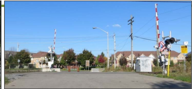
An example of a level crossing with controls
