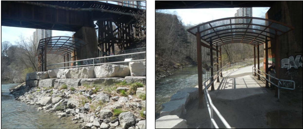
Figure 8-13: Rail line underpass along the existing East Don Trail
