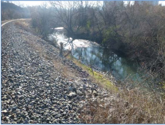
7. East Slope along CN rail.
