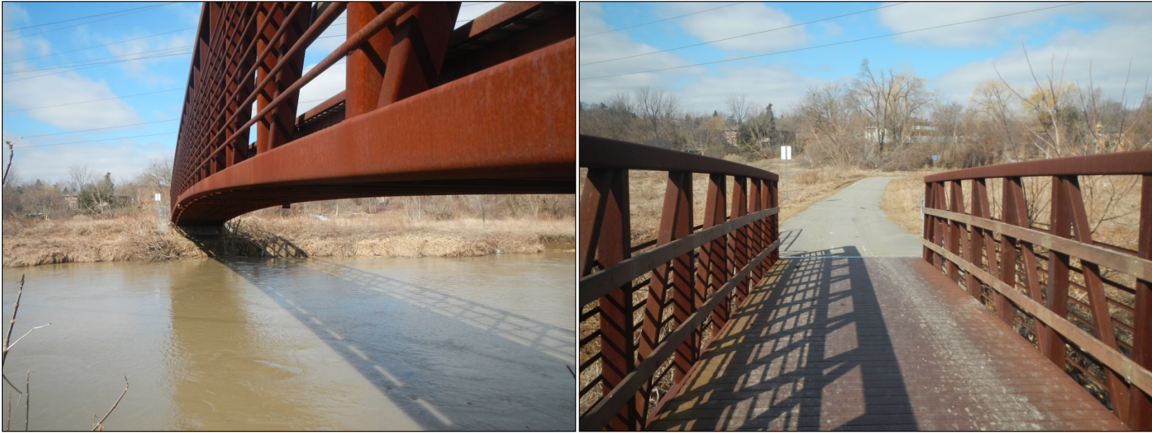
Figure 8-10: Example of weathering steel (COR-TEN) prefabricated bridge along the Humber River
