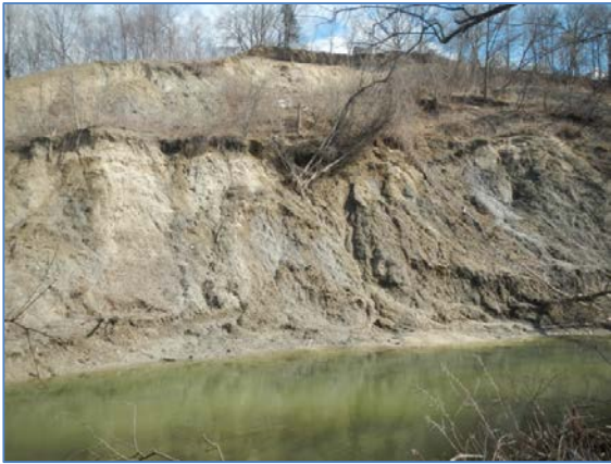
9. East Slope along City Northline property.
