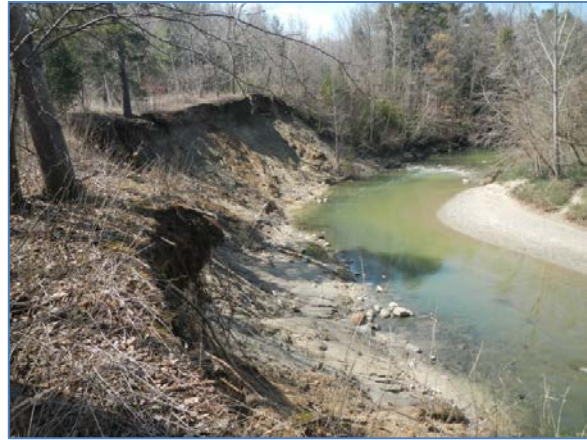
4. West Slope at base of CN Rail.
