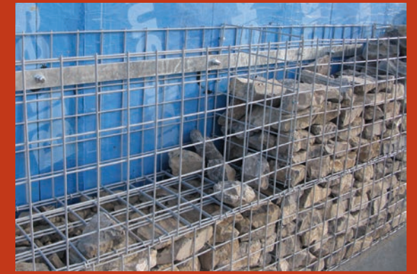
NARROW GABION WALL CONSTRUCTION
