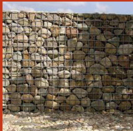
FIELDSTONE GABION WALL
