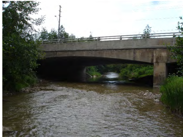
Upstream of Concrete Bridge
