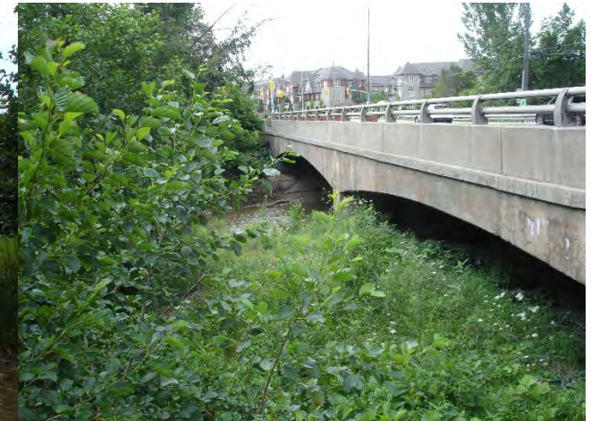
Downstream of Concrete Bridge
