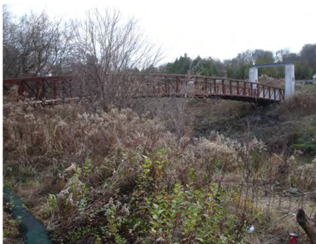
Upstream of Pedestrian Bridge
