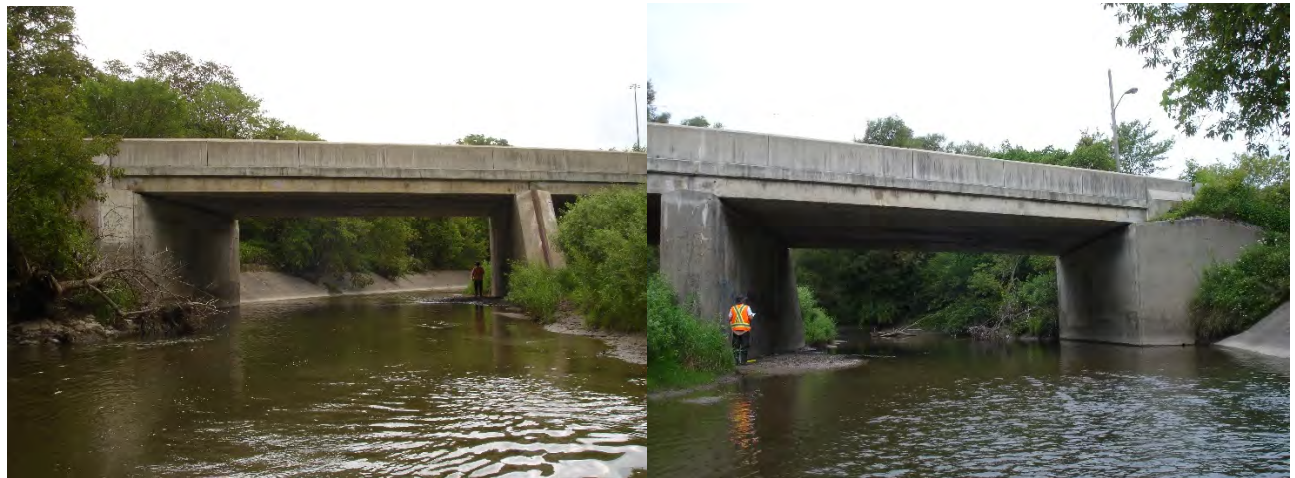
Upstream of Concrete Bridge
