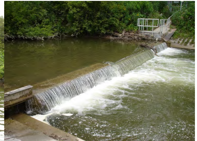
Downstream of Concrete Weir
