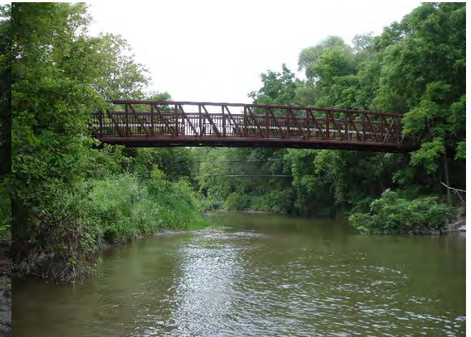
Downstream of Pedestrian Bridge
