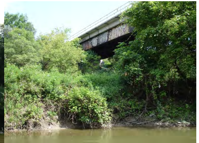
Downstream of Go Transit Bridge
