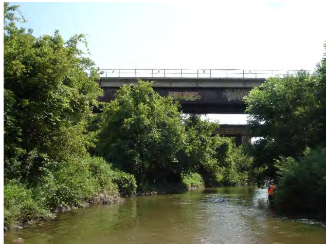
Upstream of Go Transit Bridge
