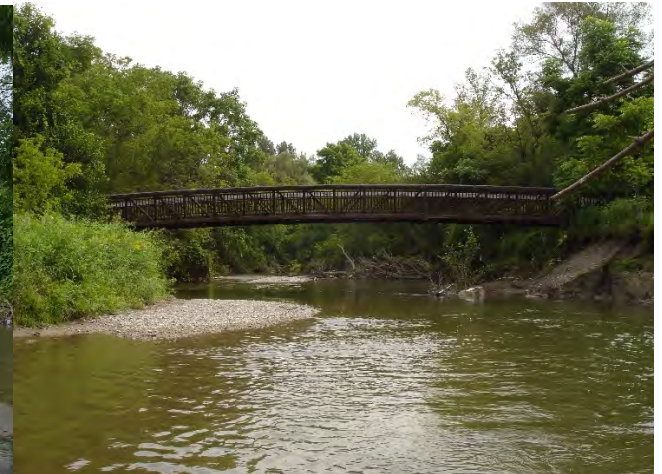
Downstream of Pedestrian Bridge
