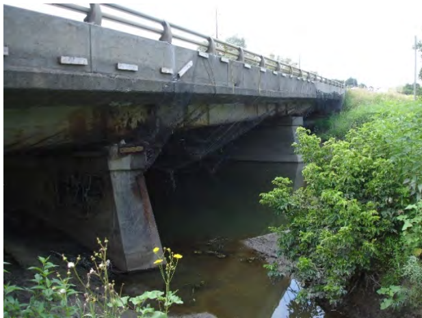
Upstream of Concrete Bridge
