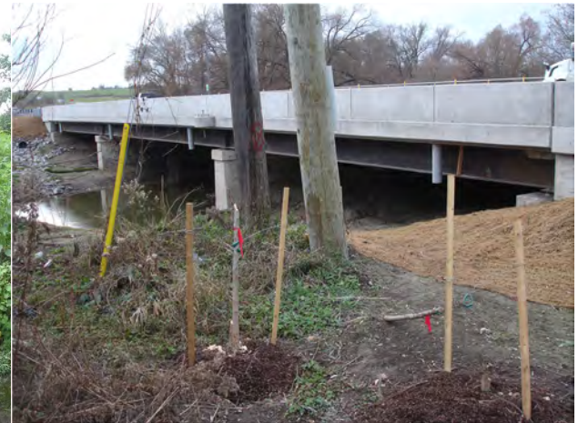
Downstream of Concrete Bridge
