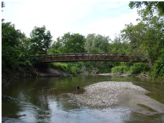
Upstream of Pedestrian Bridge
