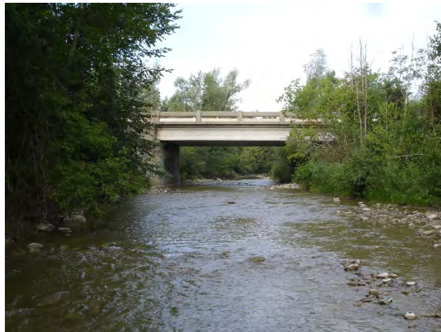
Downstream of Concrete Bridge
