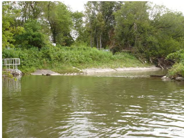
Upstream of Concrete Weir
