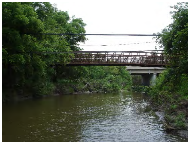
Upstream of Pedestrian Bridge
