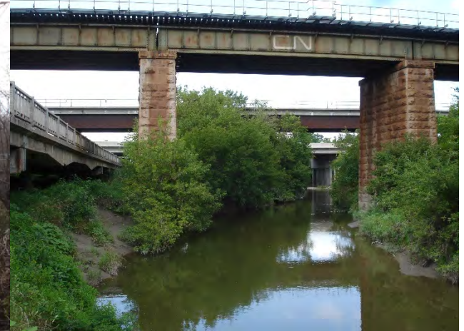
Downstream of CN Rail Bridge
