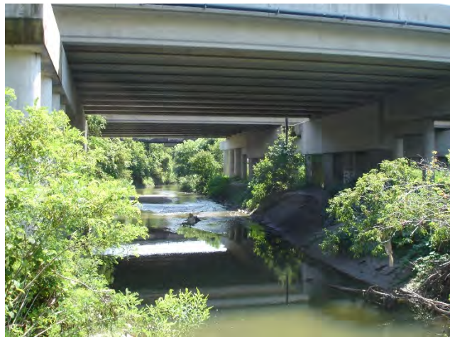
Upstream of HWY 401 Bridge
