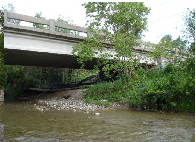
Downstream of Concrete Bridge
