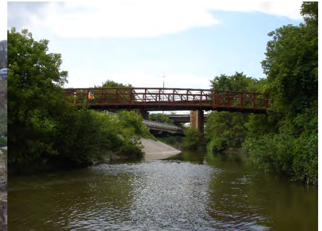
Downstream of Pedestrian Bridge
