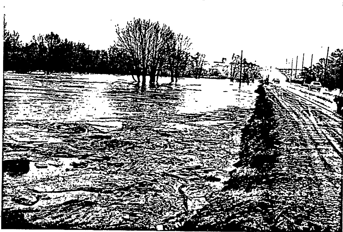
7. FLOODING AT BAYLY STREET LOOKING EAST
