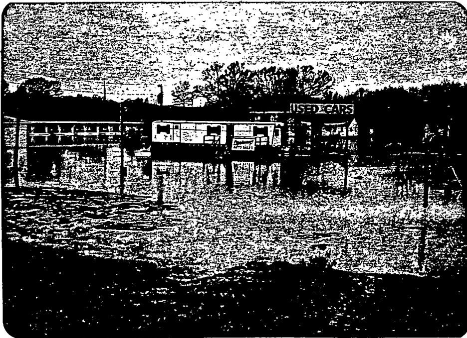
20. FLOODING AT STRUCTURES 37, 38 and 39
