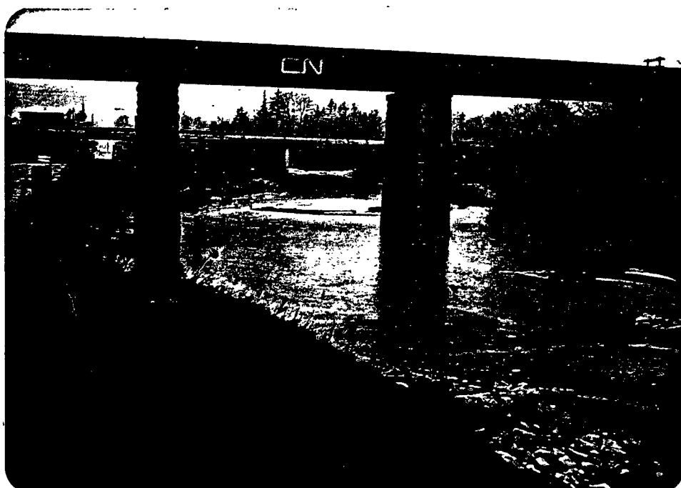
24. FLOODING AT CNR OVERPASS, LOOKING NORTH
