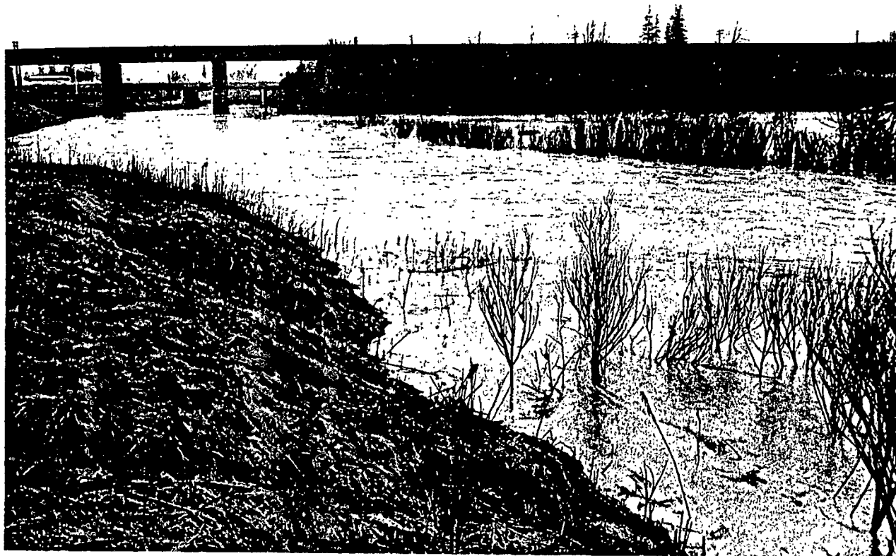
1. FLOODING AT CNR DUFFIN CREEK BRIDGE, LOOKING NORTH Photo Courtesy The News Advertiser
