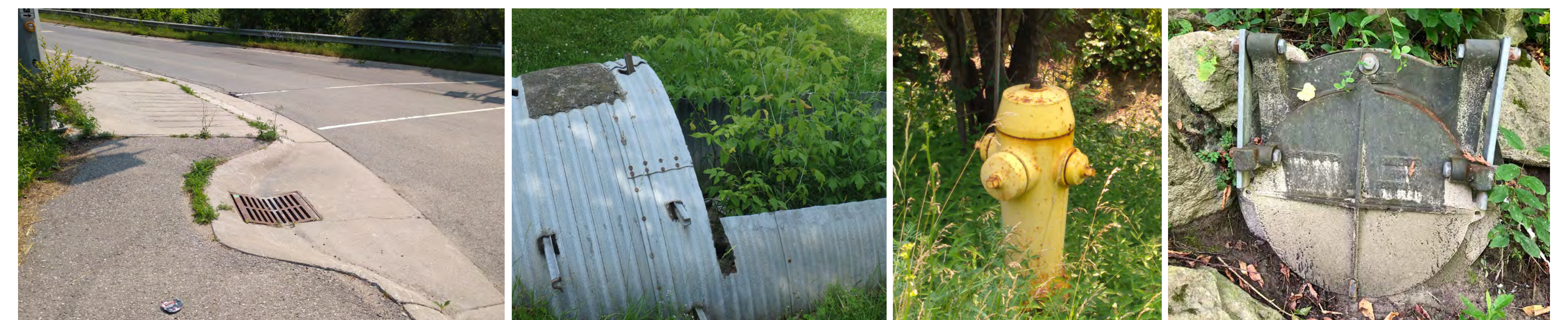
Utilities and drainage infrastructure
