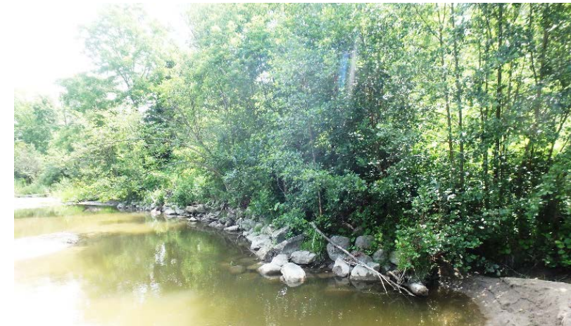
Creek bank erosion repair.
