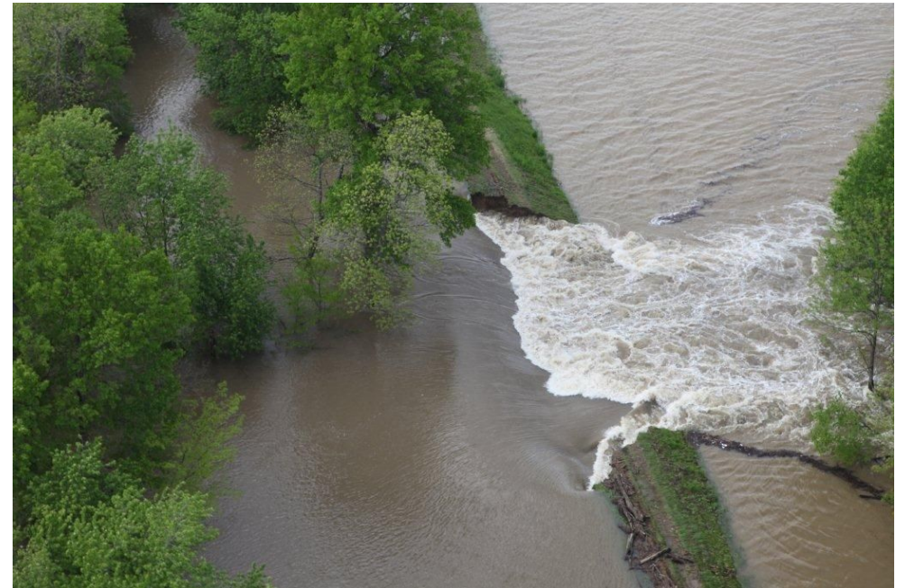
Example of a dyke failure
