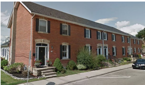
14 Church Street, Halton Hills SOURCE: GOOGLE STREETVIEW
