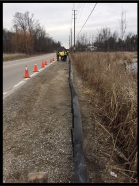
FIGURE 7. TEMPORARY FENCING INSTALLED ALONG HEART LAKE ROAD.
