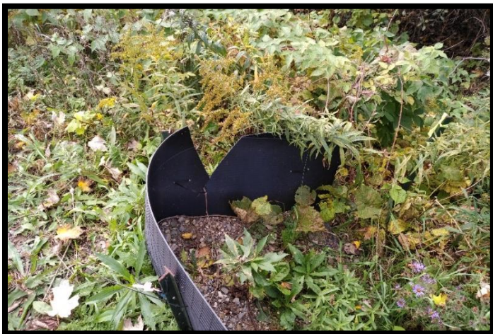
FIGURE 8. TEMPORARY WILDLIFE DIRECTIONAL FENCING END CURL.
