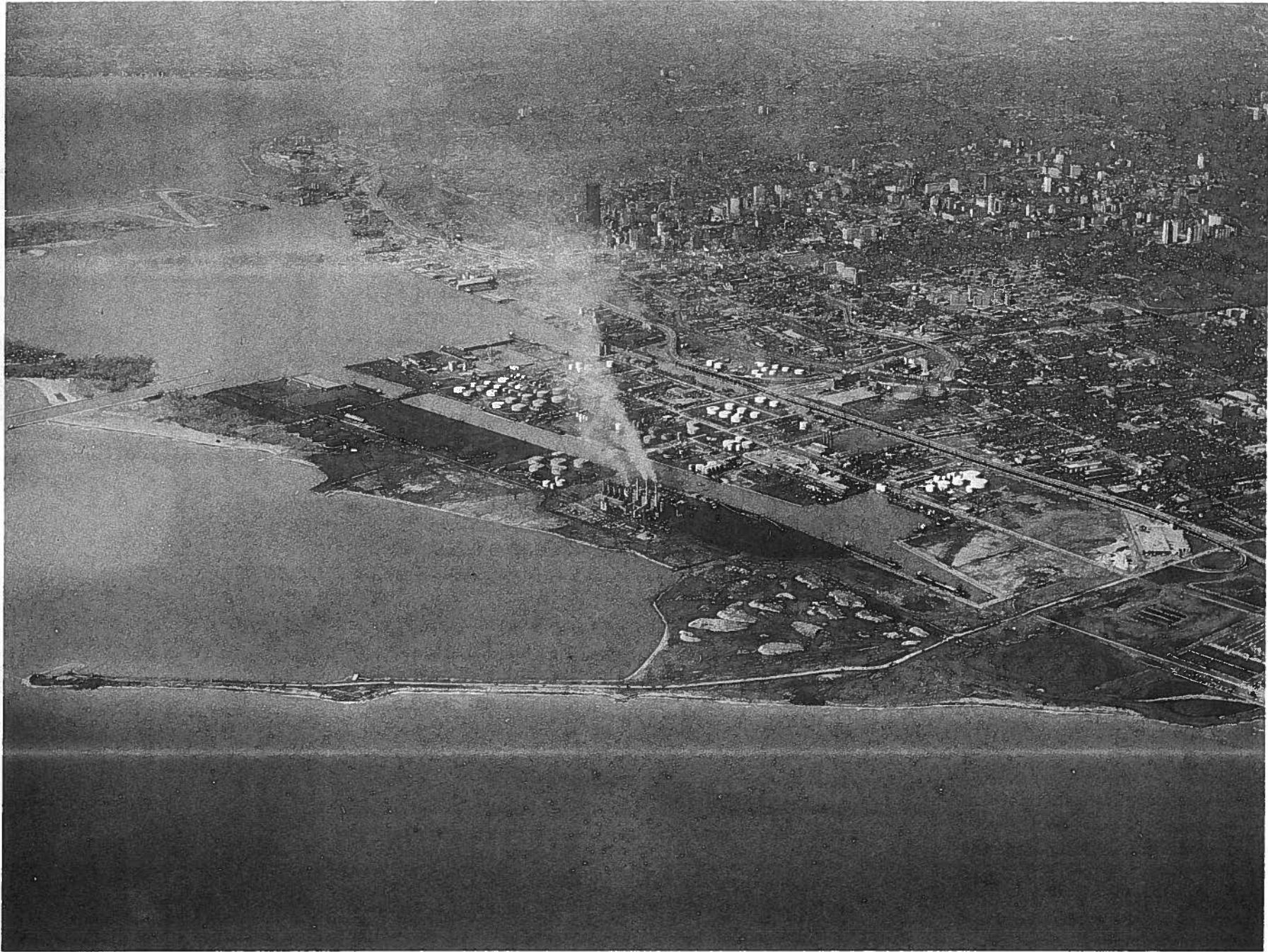
The Outer Harbour headland under construction, November 1967.
