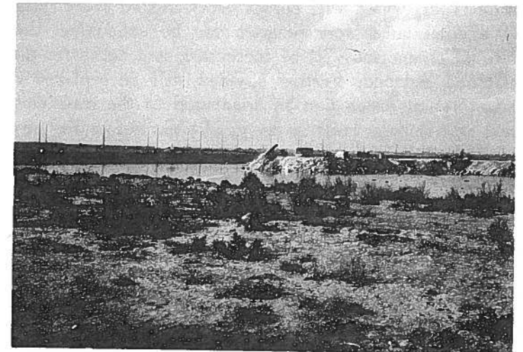
Land filling -- Port of Copenhagen
