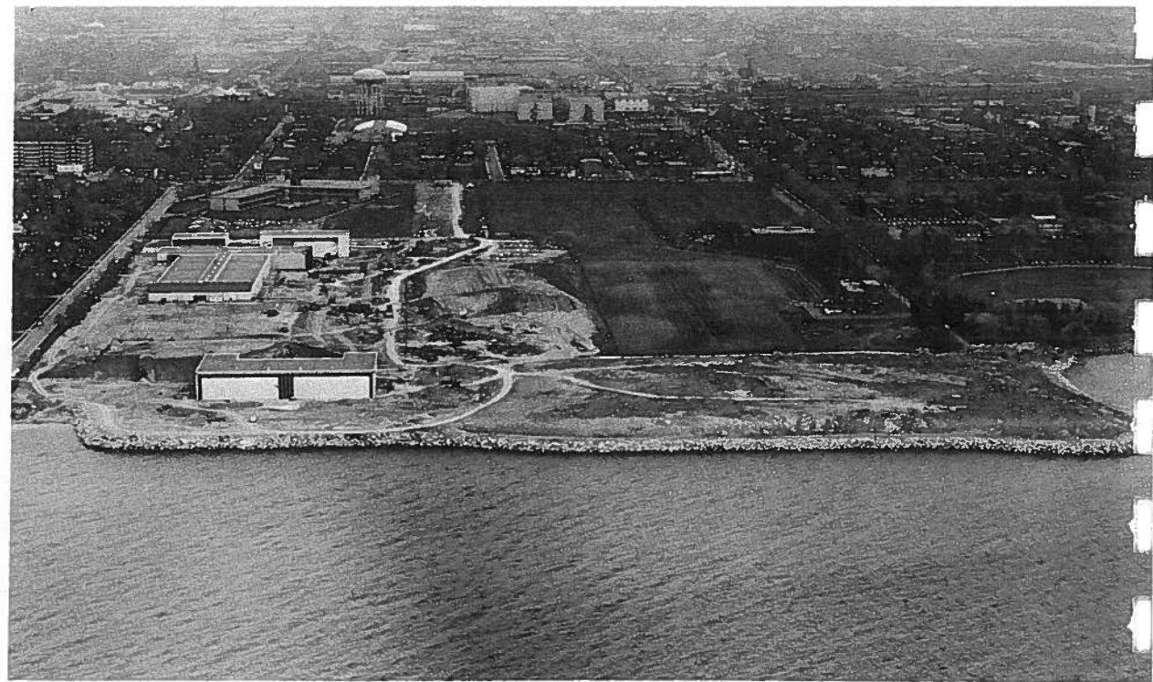
The Westerly Water Filtration Plant under construction and the Ontario Hospital grounds, New Toronto.
