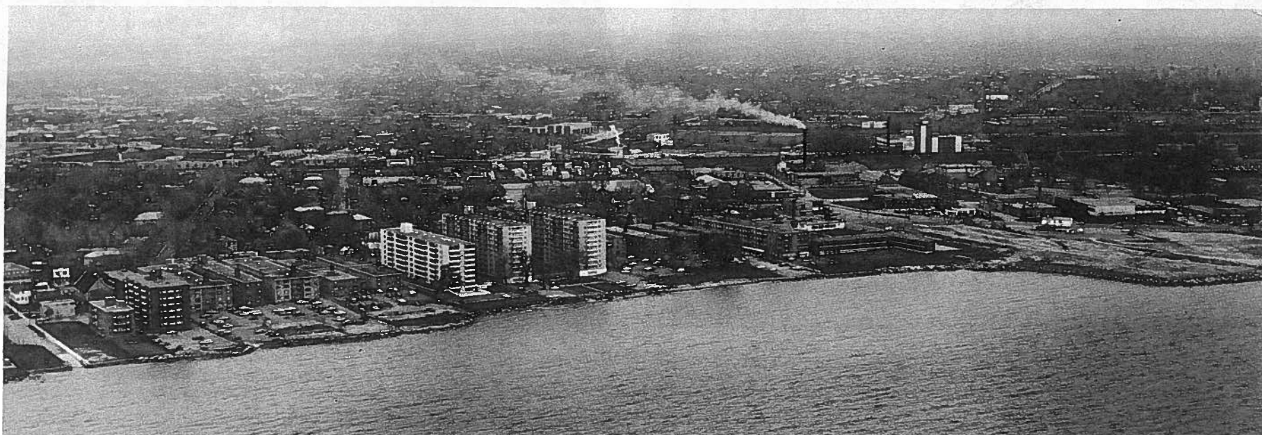
Apartment development in Mimico has taken little advantage of the lakefront setting. Private lake filling at right.
