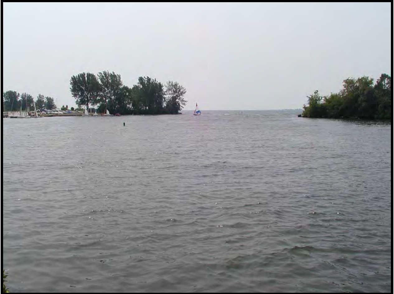
Plate 9: Coatsworth Cut looking South
