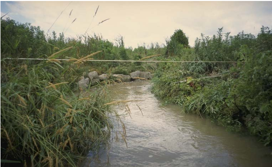
Photo 2. At monitoring cross-section looking upstream.
