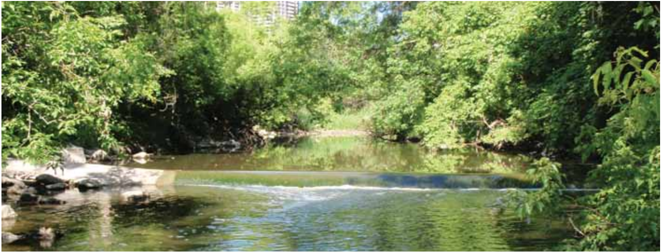
Fish Barrier north of Meadowvale Drive
