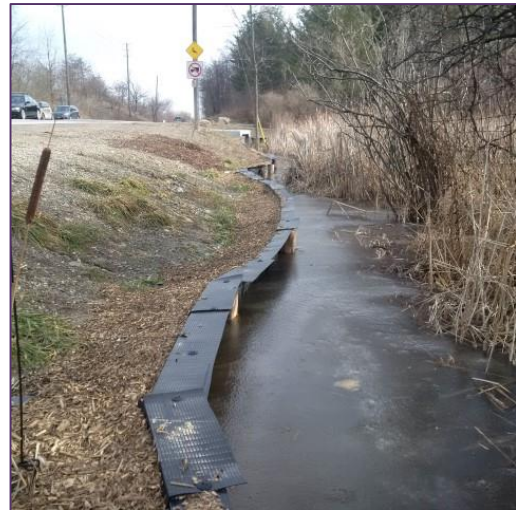
Figure 18: Animex fencing banked with mulch leading to passage
