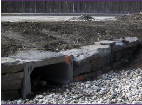
Figure 5: Wildlife passage/fence, Terry Fox Dr, City of Ottawa (Photo courtesy of Dillon Consulting Ltd)
