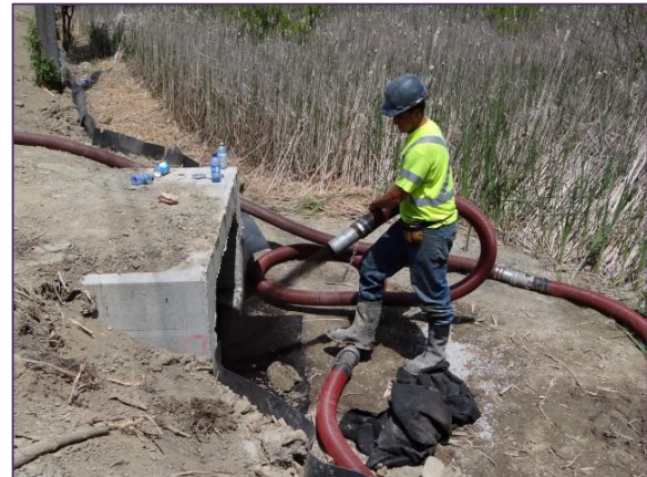
Figure 16: Soil/mulch substrate being "blown" into passage
