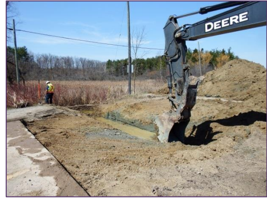
Figure 14: CoB digs trench at Heart Lake Road to install passage
