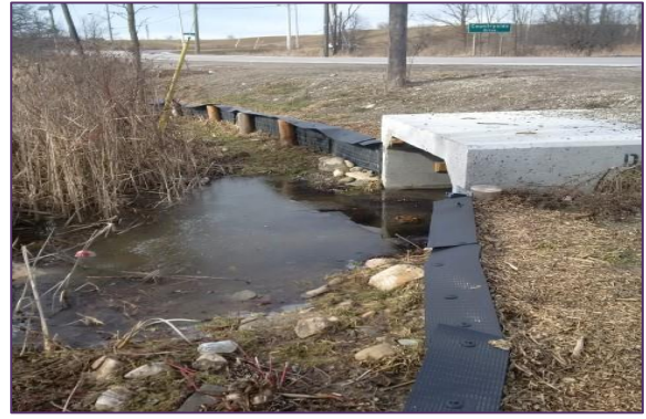
Figure 12: Dedicated wildlife passage and wildlife directional fencing
