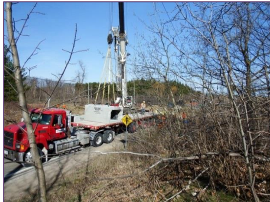
Figure 15: Oversized concrete culvert sections at site
