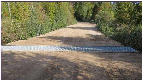
Figure 1: Bruce Peninsula National Park ecopassage (Photo courtesy of Parks Canada)
