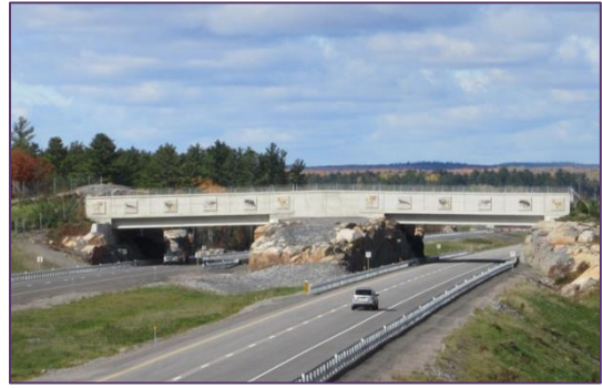
Figure 4: MTO wildlife overpass Hwy #69 (Photo courtesy of Ministry of Transportation Ontario)
