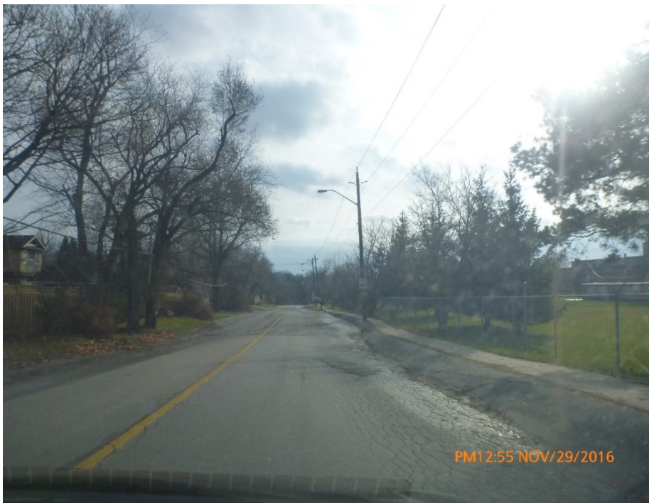
Southbound Brimley Road, south of Kingston Road (Source: WSP, November 29, 2016)
