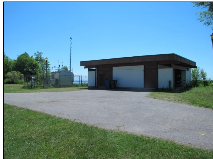
Image 4 Existing structure and roadway facing southeast
