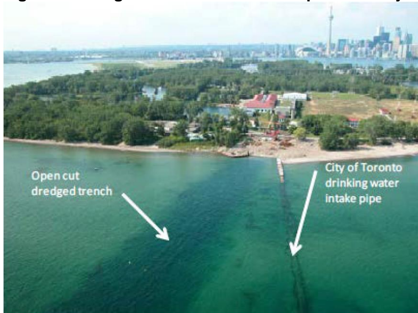
Figure 4: Dredged Trench and Intake Pipe near Project Area
