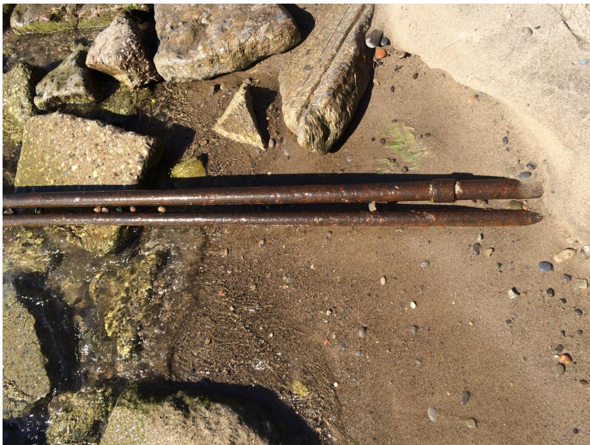
Figure 30 – Pipeline Extending from Shore
