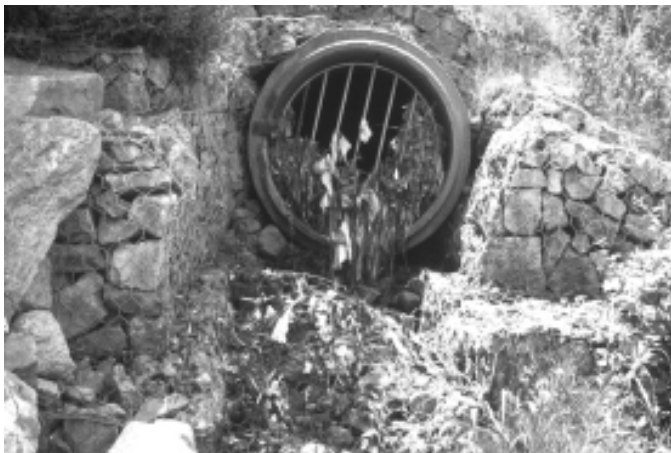
Stormsewer outfall discharging into the Highland
