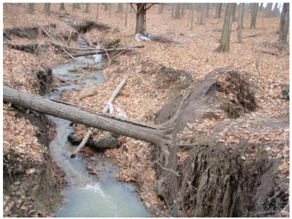
**FIGURE 4**: Duke of Richmond, Richmond Hill. Shows the erosion problems that exist at this site downstream of the stormwater pond outlets. Note the exposed roots and fallen trees. Prior to development upstream, the bankfull depth of the watercourse was approximately 0.2-0.3 m. Now the bankfull depth is 2-3 m.
