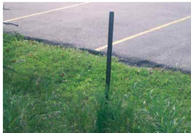
2. Fence down along boundary with Meadowbrook Golf & Country Club
