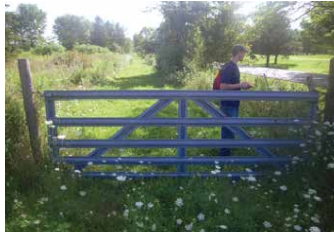
12. Service gate next to Meadowbrook Golf & Country Club, along Warden Ave.
