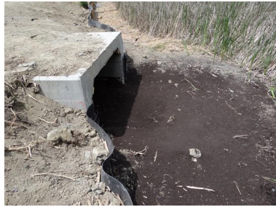
Figure 20 - Soil/mulch substrate extending beyond passage entrance
