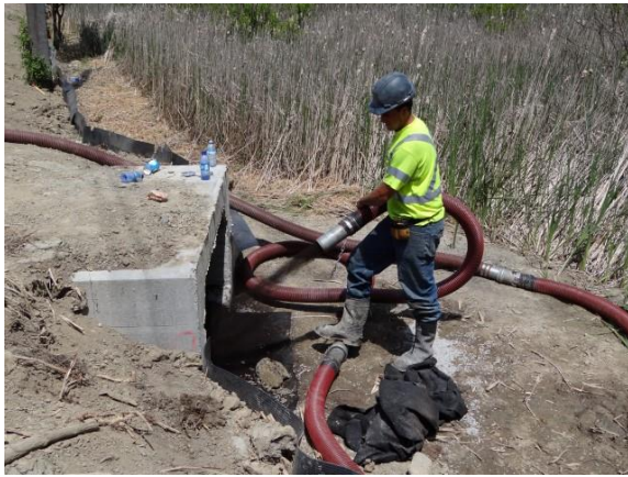
Figure 19 - Soil/mulch substrate being "blown" into passage
