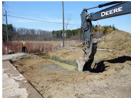
Figure 16 - CoB digs trench at Heart Lake Road to install passage
