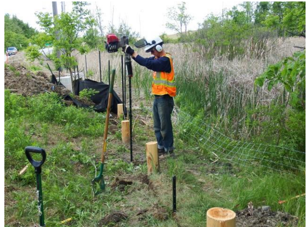
Figure 25 - Installation of steel T-bars for reinforcement
