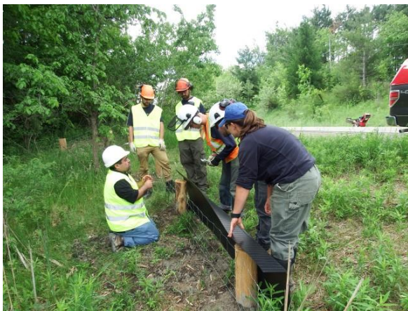
Figure 26 - TRCA staff install Animex fencing to poles
