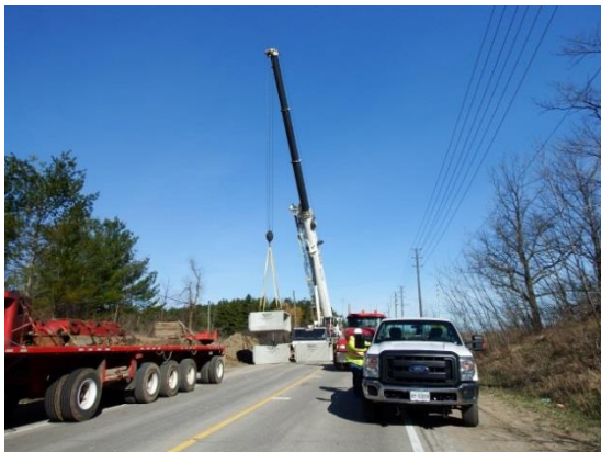
Figure 17 - Oversize concrete culvert sections craned to site
