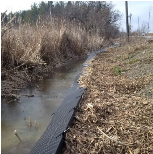
Figure 28 - Animex fencing banked with mulch
