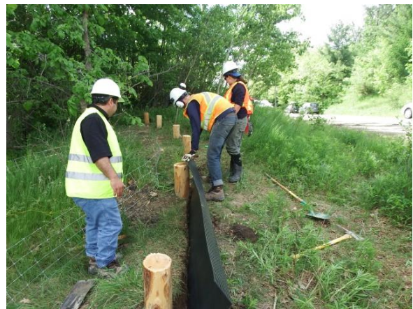
Figure 27 - TRCA staff install Animex fencing
