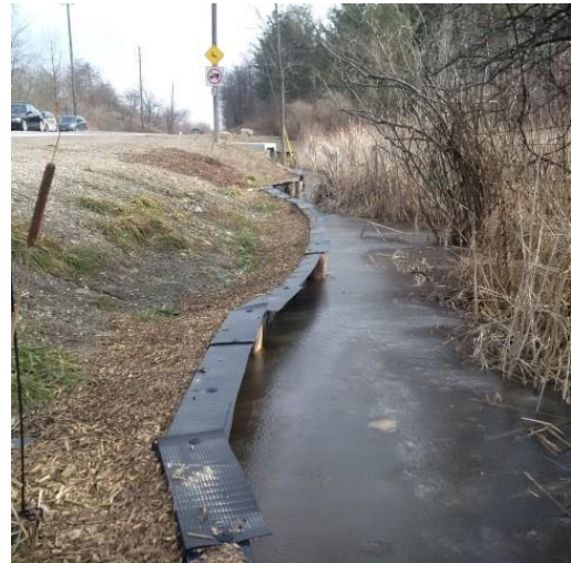
Figure 29 - Animex fencing banked with mulch leading to passage
